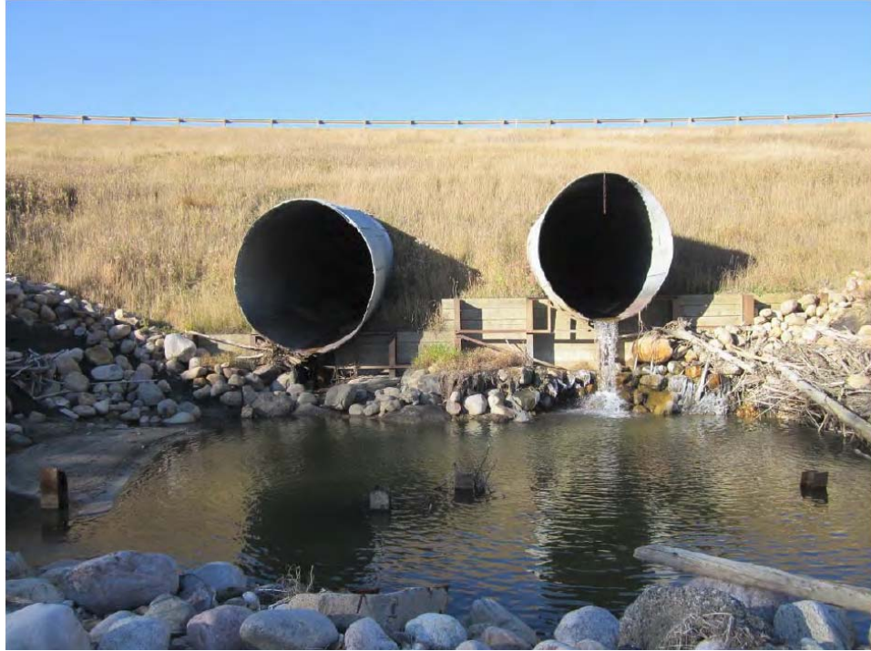
Looking at outlets from Downstream (note ~2m drop, scour hole)
