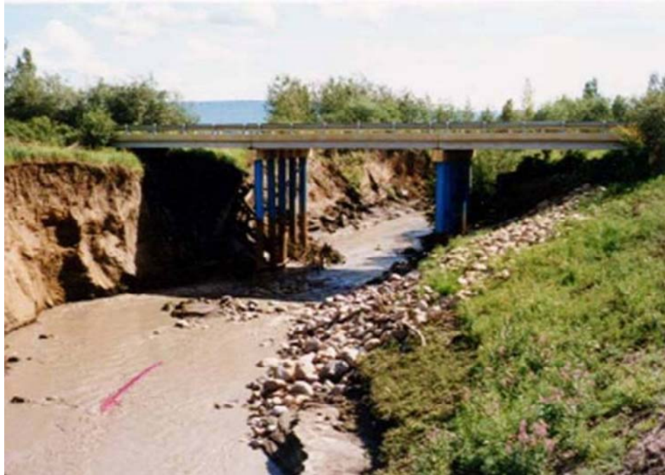
1987 Photo: note paint elevation and vertical banks
