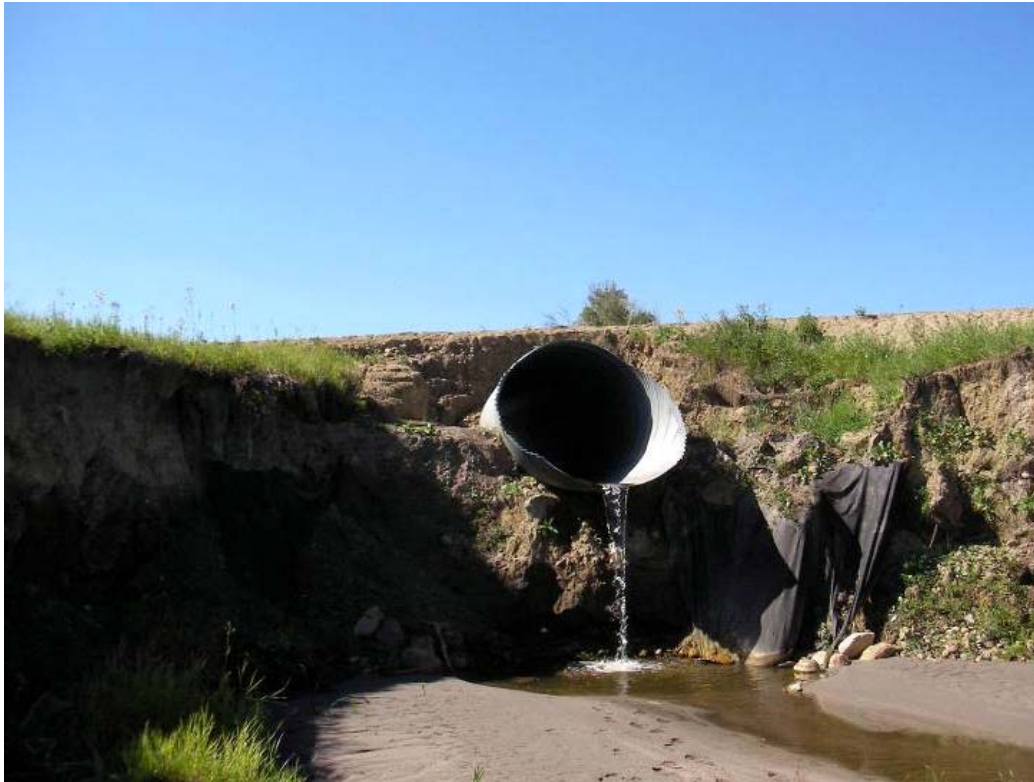
2007 Photo – note hanging outlet, vertical banks
