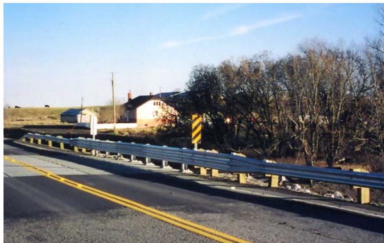
Figure 5.10 PL1 Thrie Beam Bridgerail without Curb
