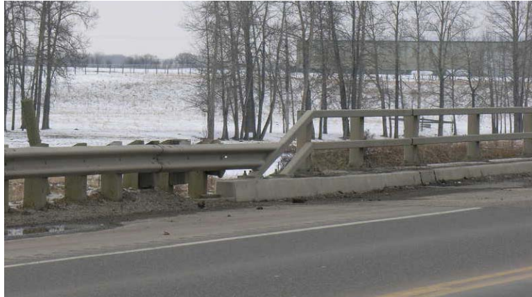
Figure 5.16 Flexbeam attached to Double Tube Bridgerail
