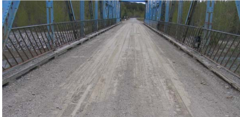
Figure 5.4 Lattice Panel Bridgerail
