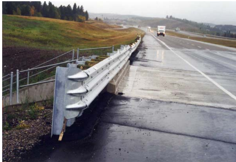
Figure 5.11 PL2 Thrie Beam Bridgerail on Concrete Curb
