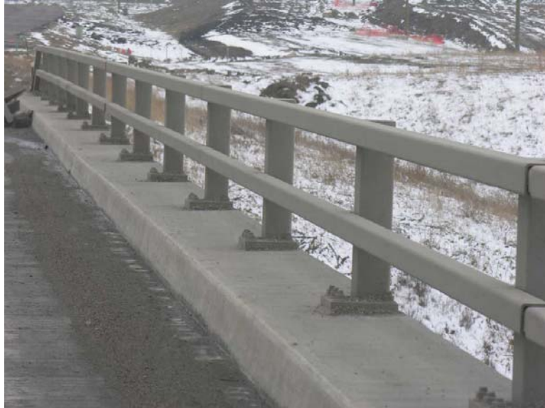
Figure 5.6 Double Tube Bridgerail on Safety Curb
