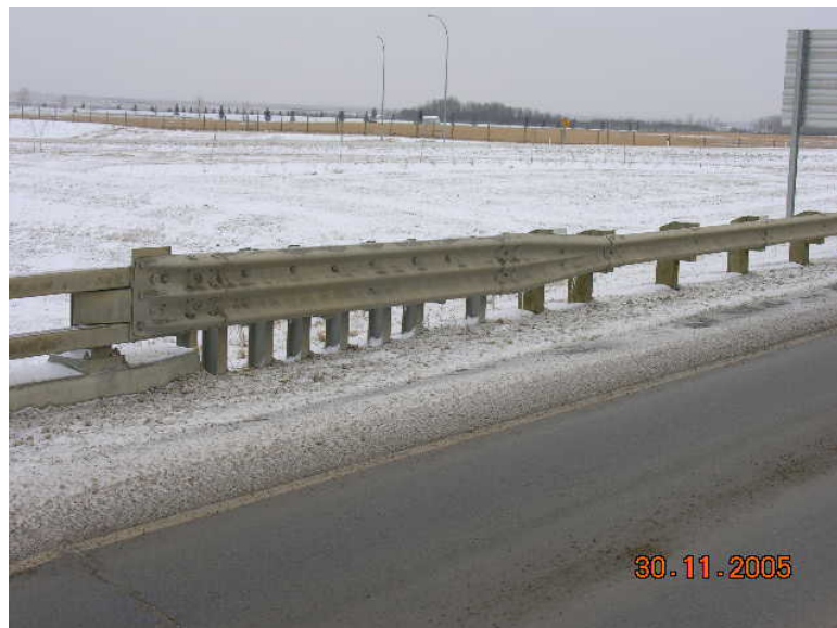
Figure 5.17 PL2 Approach Transition Section
