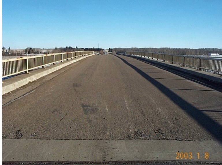
Figure 5.2 Vertical Steel Bar Bridgerail
