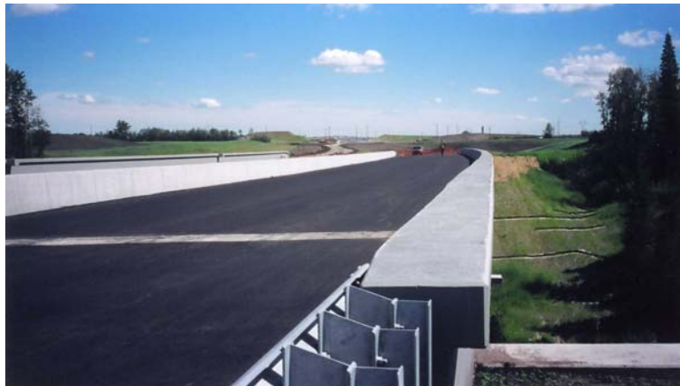
Figure 5.13 PL2 Concrete Barrier Bridgerail
