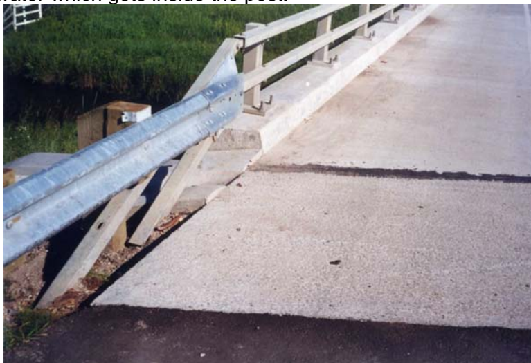
Figure 5.7 Double Tube Bridgerail on Standard Prestressed Girders with Soil Anchors
