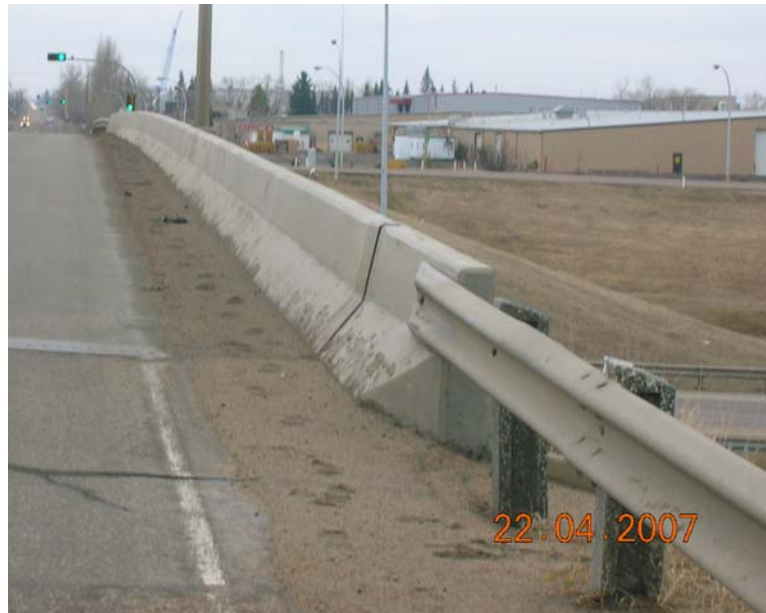
Figure 5.8 Concrete Barrier Bridgerail
