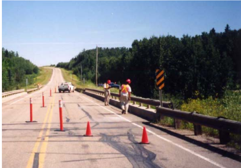
Figure 5.14 Approach Flexbeam lined up with face of curb
