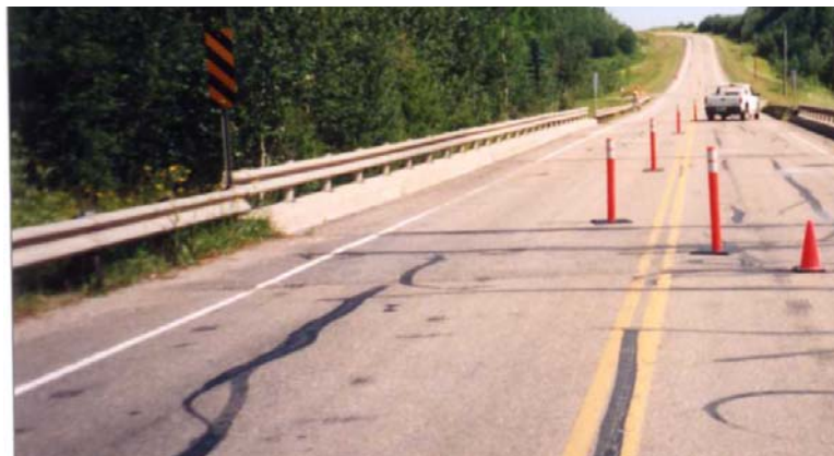
Figure 5.15 Exit Flexbeam line up with bridgerail
