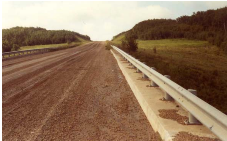
Figure 5.9 Double Layer Flex-beam Bridgerail
