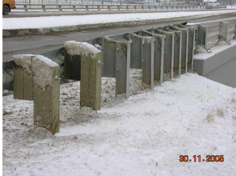
Figure 5.18 Back of PL2 Transition Section
