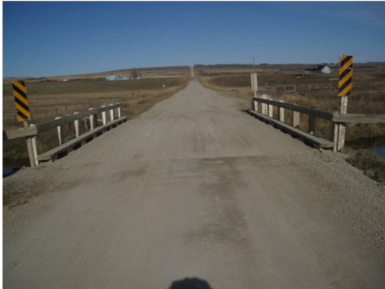
Figure 5.1 Timber Bridgerail
