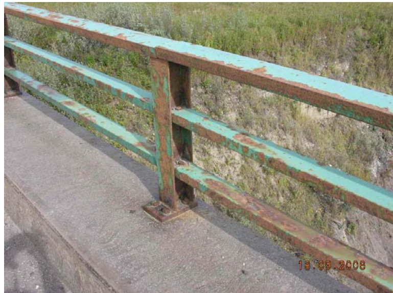
Figure 5.3 Horizontal Steel Rail Bridgerail
