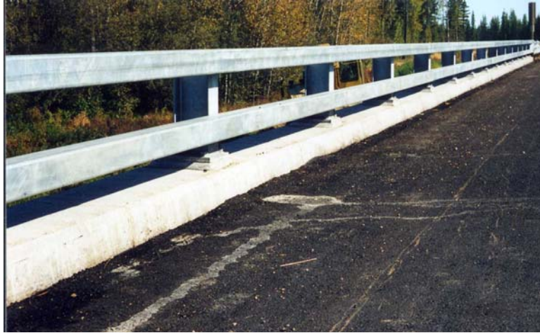
Figure 5.12 PL2 Double Tube Bridgerail
