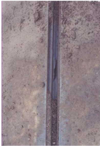
Figure 6-7 Torn seal
