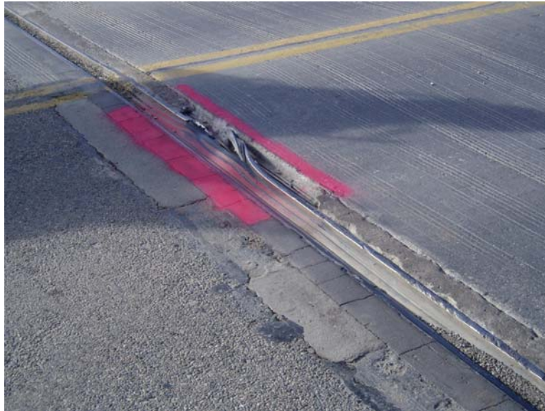
Figure 6.9 Damage to metal extrusion
