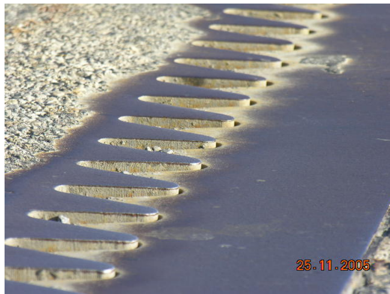
Figure 6-3 Vertical misalignment of finger joint
