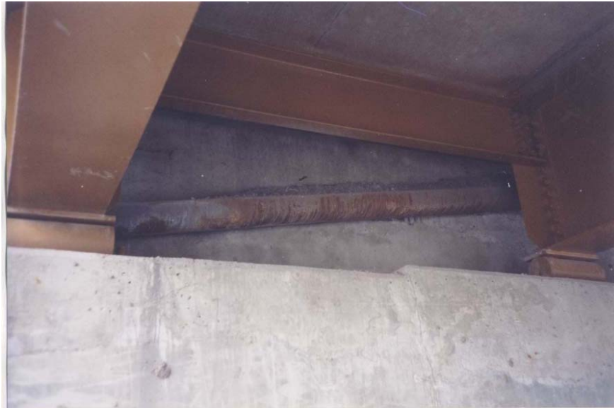
Figure 6-6 Drain filled with sand and starting to corrode
