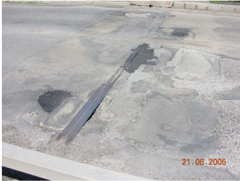
Figure 6.11 Deterioration of concrete at buffer angles
