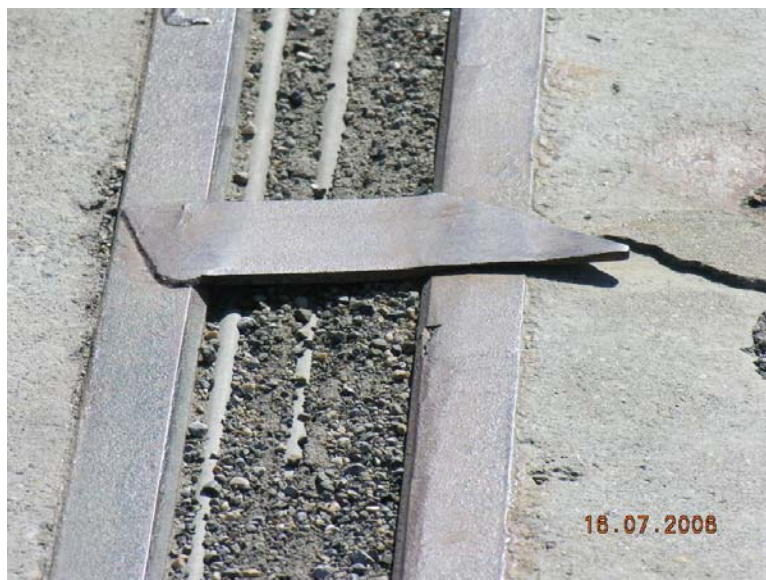
Figure 6.10 Damaged snow plow guard
