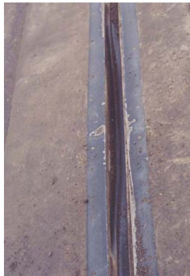
Figure 6-8 Dislodged seal
