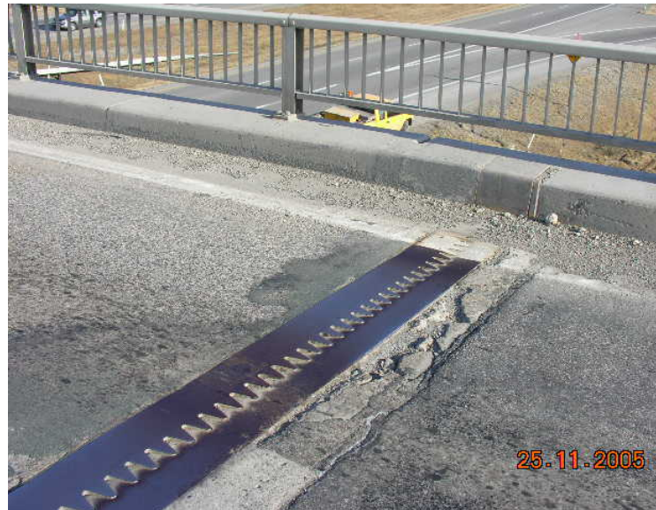
Figure 6-4 Deterioration of concrete paving lip
