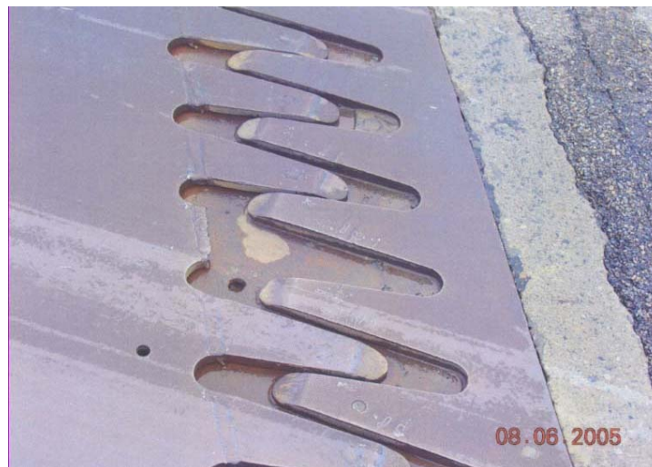
Figure 6-5 Fingers not properly aligned and broken finger
