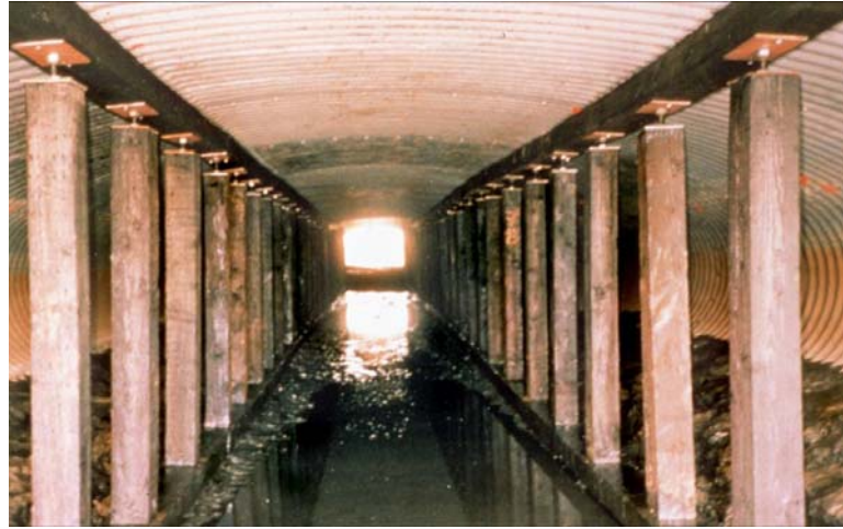
Figure 7-11 Strutting
