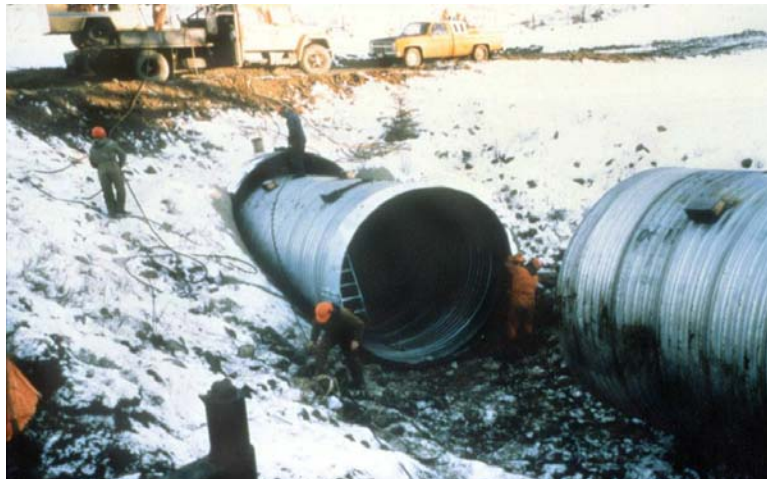
Figure 7-13 Culvert liner
