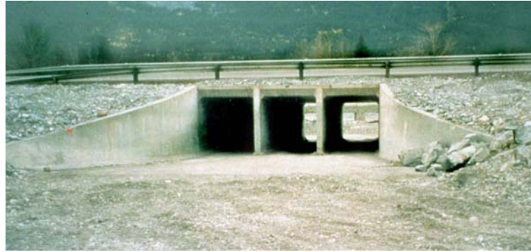
Figure 7-1 Concrete Box Culvert
