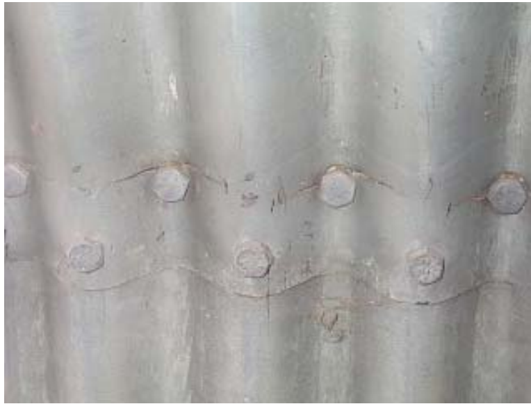
Figure 7-7 Cracking of plate between bolt holes
