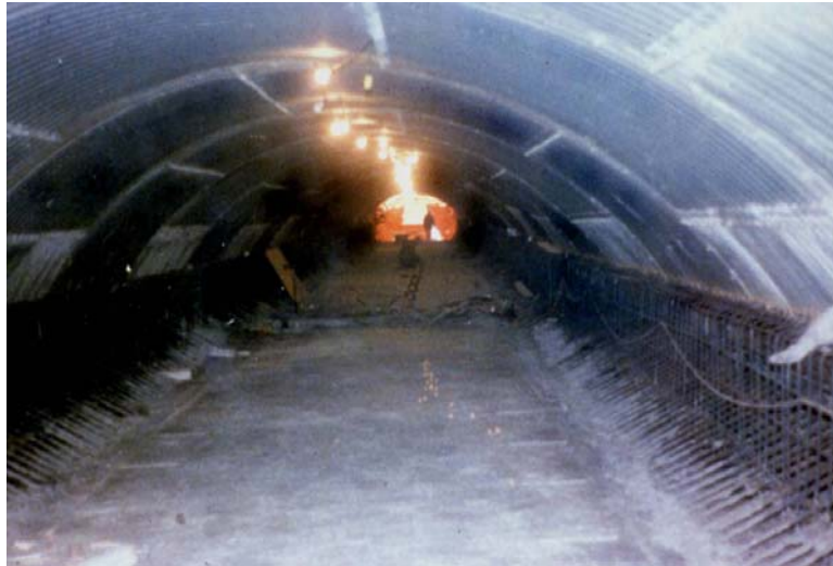
Figure 7-14 Concrete floor with partial concrete walls
