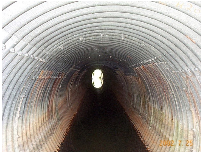
Figure 7-9 Corrosion due to soil
