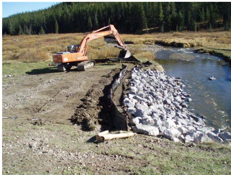
Figure 7-16 Scour repair
