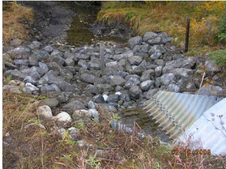
Figure 7-15 Rock Rip Rap at culvert outlet
