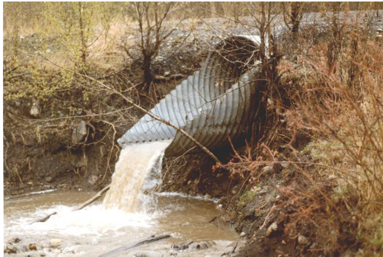
Figure 7-10 Culvert scour
