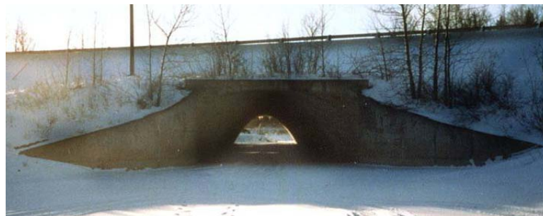
Figure 7-2 Concrete Arch Culvert
