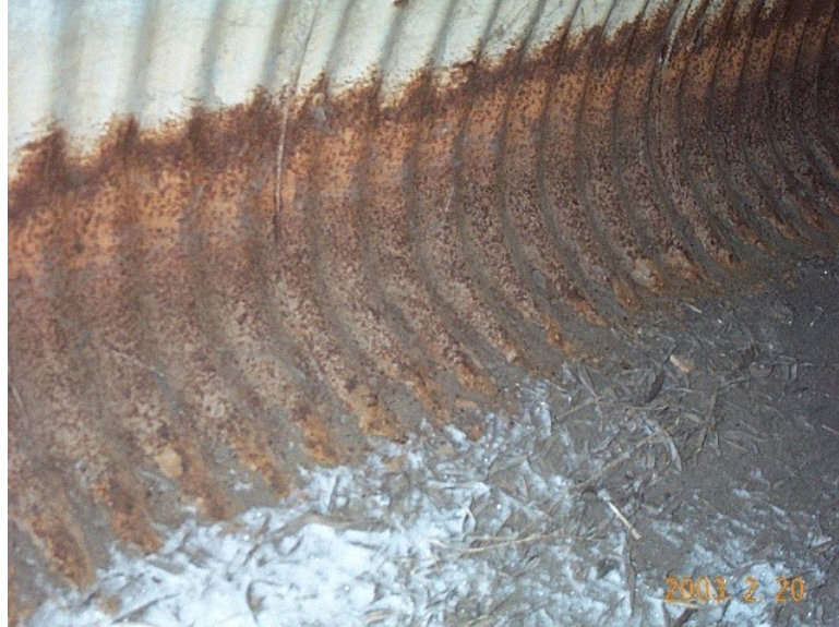
Figure 7-8 Corrosion due to water
