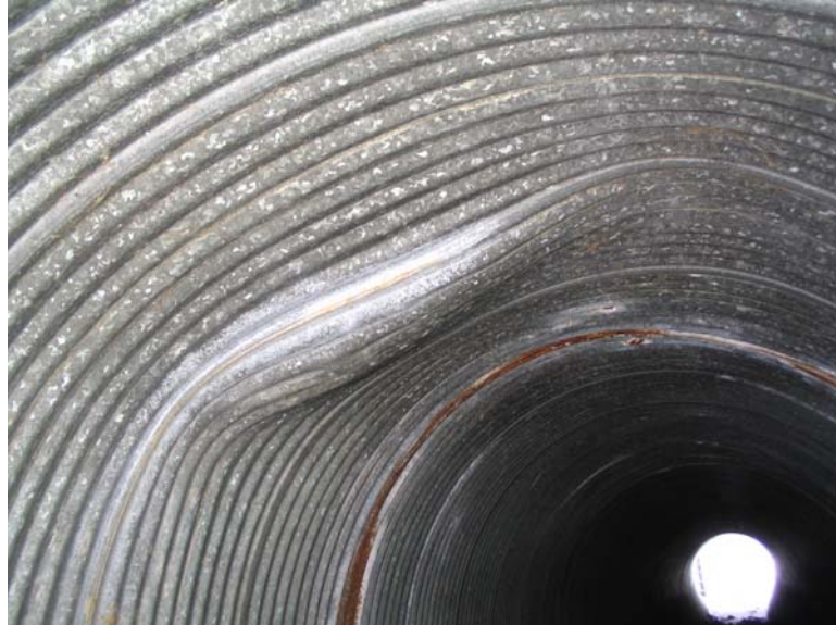
Figure 7-5 Deformation of culvert shape
