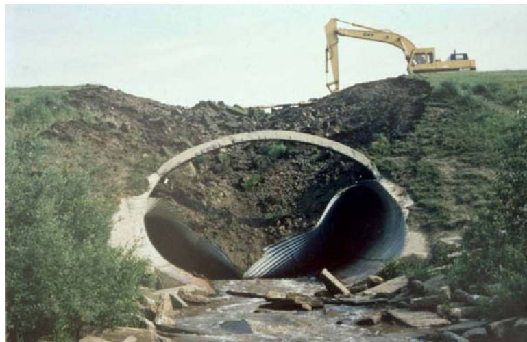
Figure 7-6 Collapsed culvert
