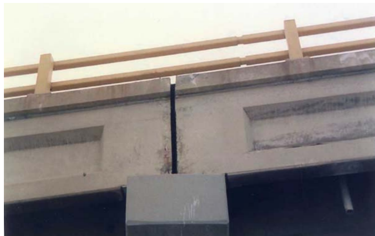
Figure 8-15 Type FC Girder – Typical vertical crack with corrosion staining at girder end
