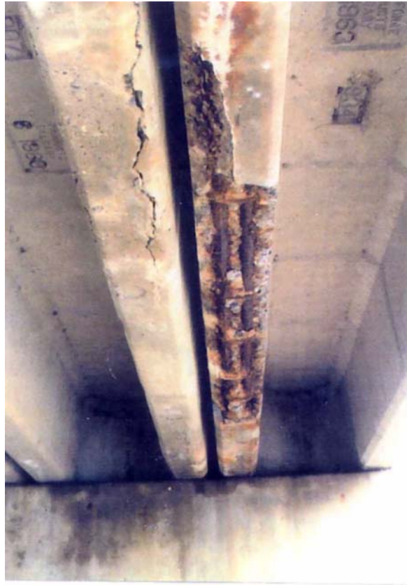
Figure 8-2 Type PE Girder – Spalling on leg of curb girder
