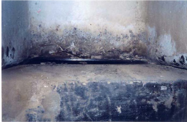
Figure 8-4 Type HC Girder – Deteriorated end diaphragm
