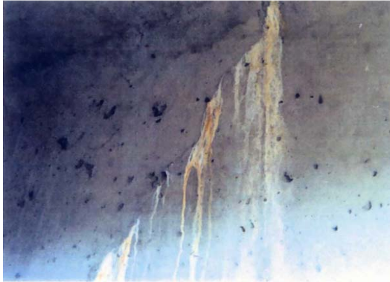
Figure 8-8 Type PE Girder – Shear crack with corrosion staining
