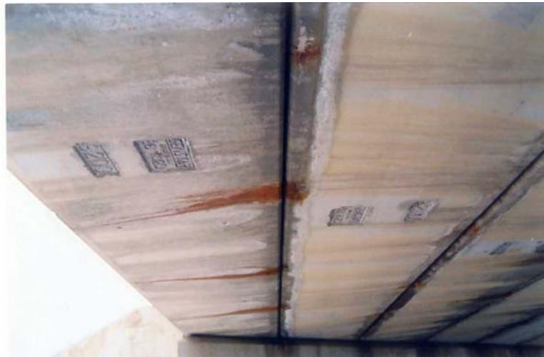
Figure 8-9 Type SM Girder – Corrosion stains from connector pockets
