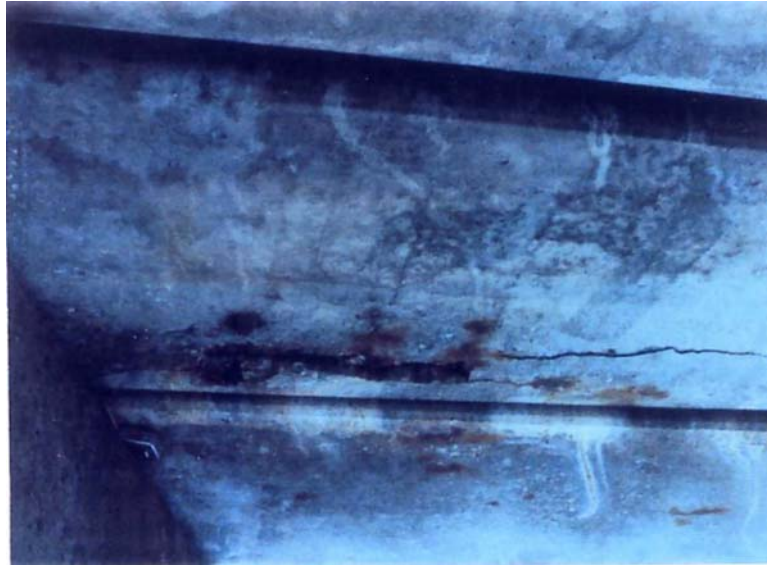
Figure 8-18 Type PM Girder – Wide crack and spall with corrosion staining at girder bottom
