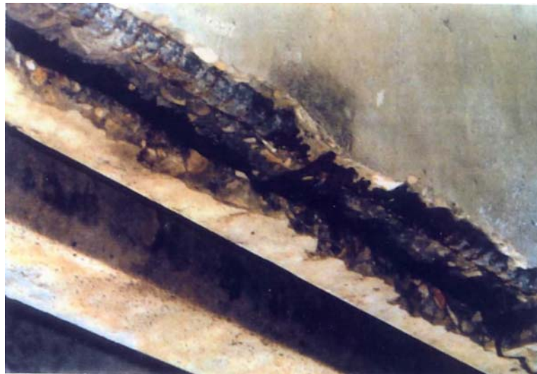
Figure 8-1 Type PG Girder – Spalling on girder leg
