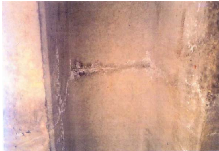
Figure 8-6 Type PE Girder – Crack along both webs and deck underside
