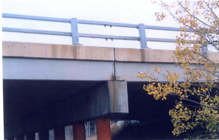
Figure 8-12 Type SM Girder – Typical vertical crack at girder end
