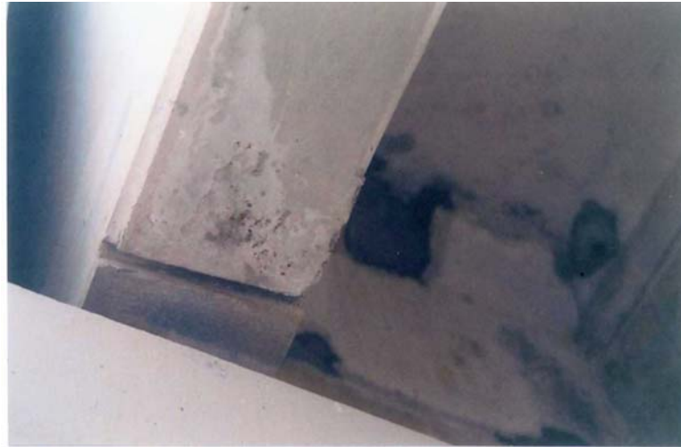
Figure 8-16 Type FC Girder – Corrosion spots on underside of leg near bearing with no significant effect on rating
