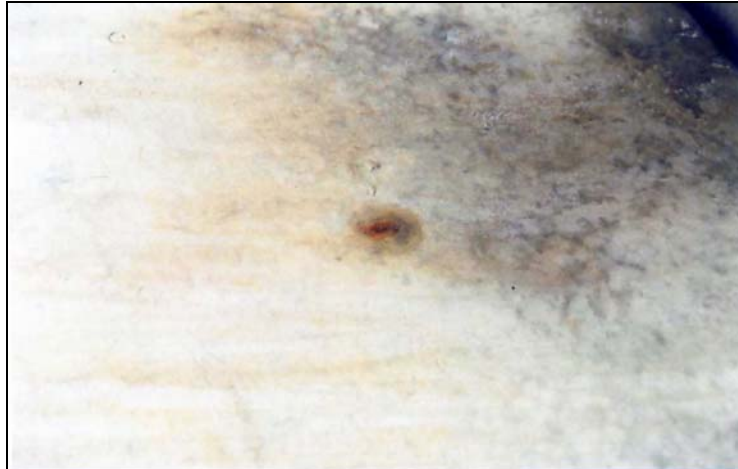
Figure 8-10 Type SM Girder – Typical corrosion spot with no significant effect on rating
