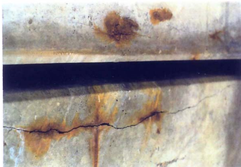
Figure 8-17 Type PM Girder – Wide crack with corrosion staining at girder bottom
