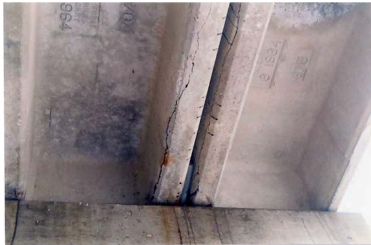
Figure 8-3 Type HC Girder – Wide crack in anchorage zone
