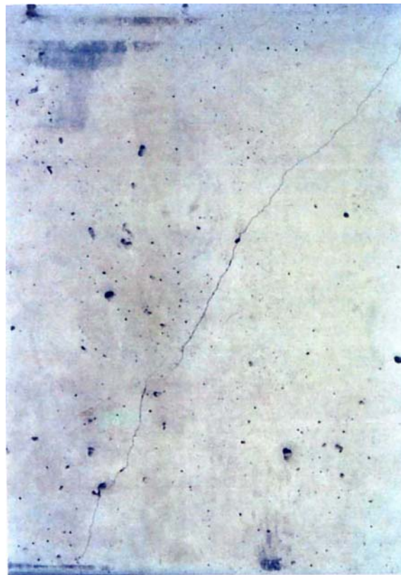
Figure 8-7 Type PE Girder – Shear crack
