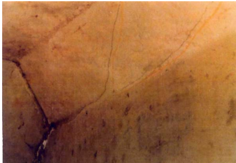
Figure 8-13 Type FC Girder – Typical crack in deck underside/web chamfer at girder end
