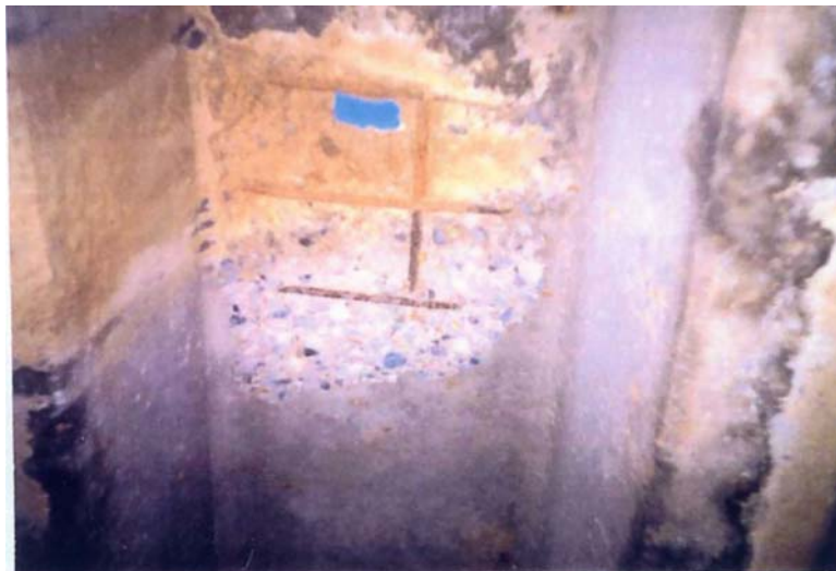
Figure 8-5 Type PX Girder – Deck punchout
