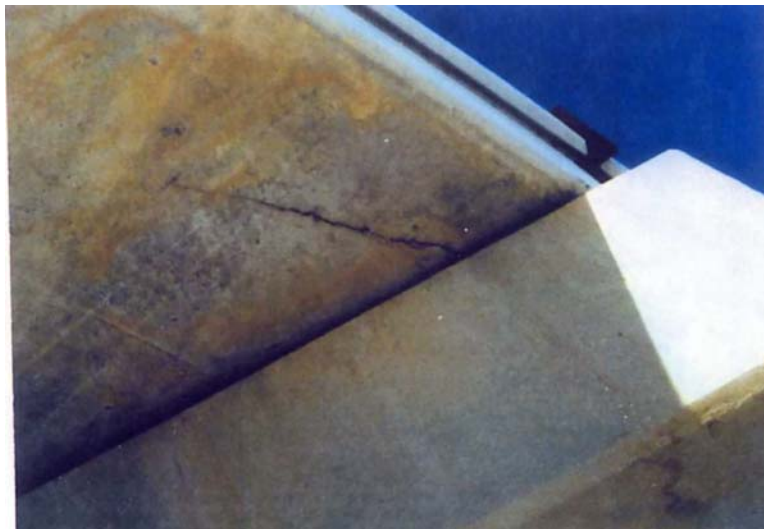
Figure 8-11 Type SM Girder – Typical diagonal crack in girder bottom at pier
