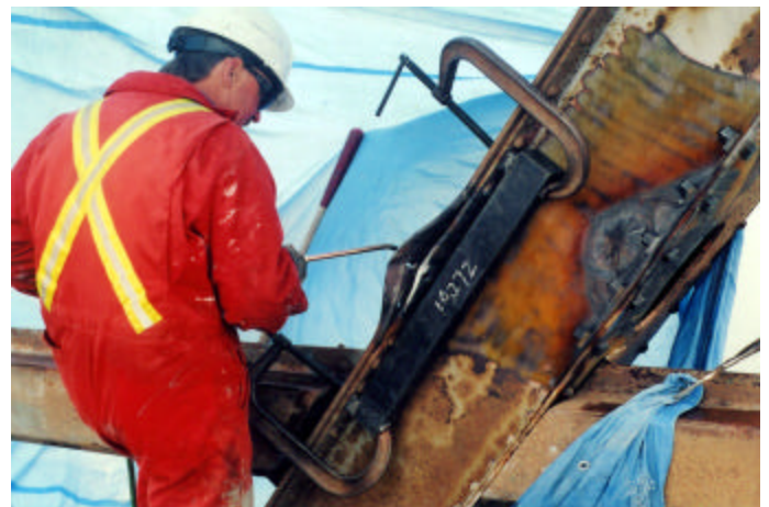
Heat straightening elements on a batterpost. Note the tarp being used to shelter from wind and cold.
