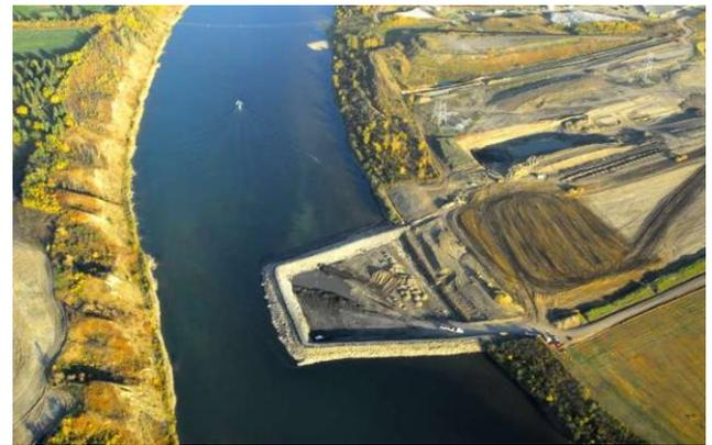
The southside river berm allows crews to build the first half of the North Saskatchewan twin bridges.
