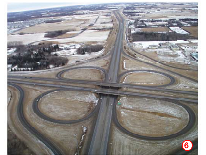
SHERWOOD PARK FREEWAY
