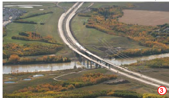
NORTH SASKATCHEWAN RIVER CROSSING
