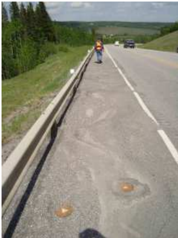
Photo S2-2 – Looking east along the pile wall area. SI#10 and AMEC BH#1 are visible in the foreground.
