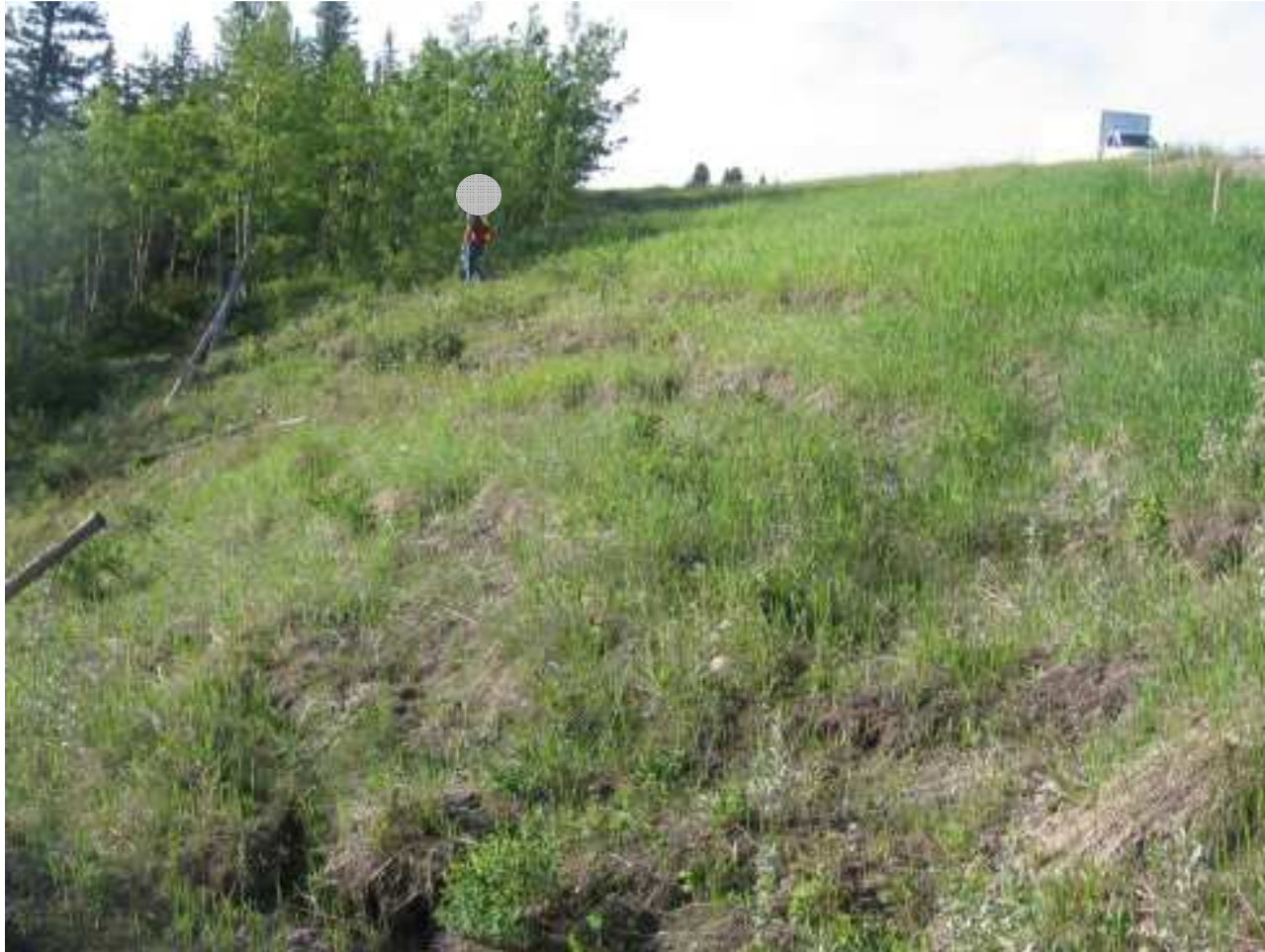
Photograph S3-5 - Looking south at the slide area below the instrumented area.
