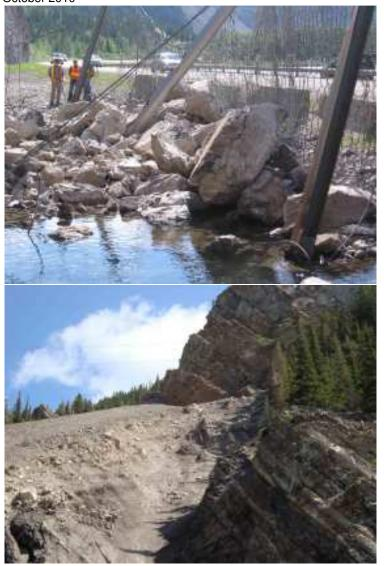
**Photo S15-4 – June 2010** Looking west along the barrier net. The large rocks are up to  $2.5 \text{ m}^3$ .
