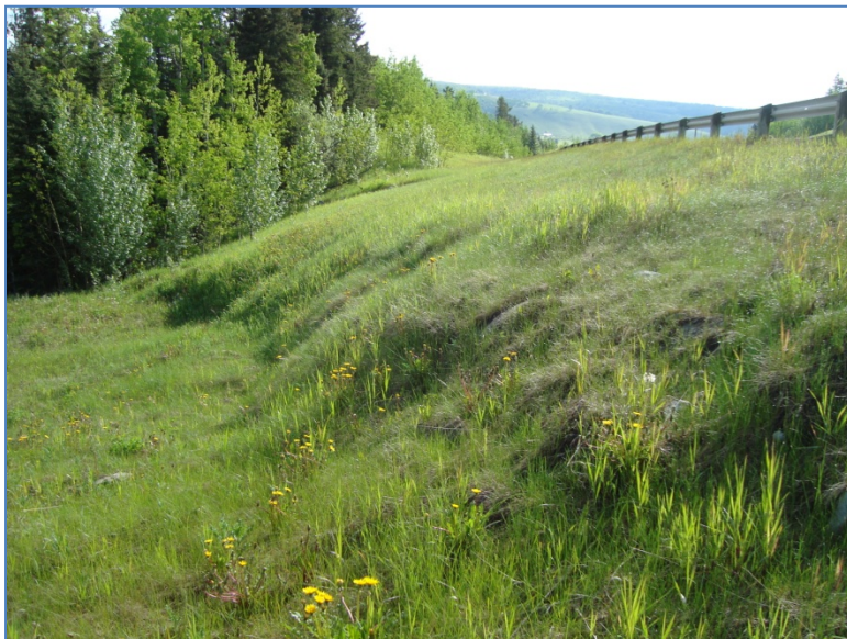
Photo S2-4 (June 2011) – Looking east at the slope below the highway in the landslide area. The slope appears to be in similar condition as was observed in 2010.
