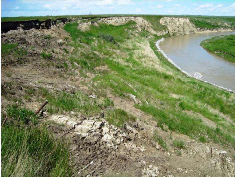
Photo S4-5 (June 2011) – Taken from near the same location as Photo S4-6. Slide movement has continued in the upper slope. The vegetation cover has become well established on the lower slope. The bank protection remains in good condition.
