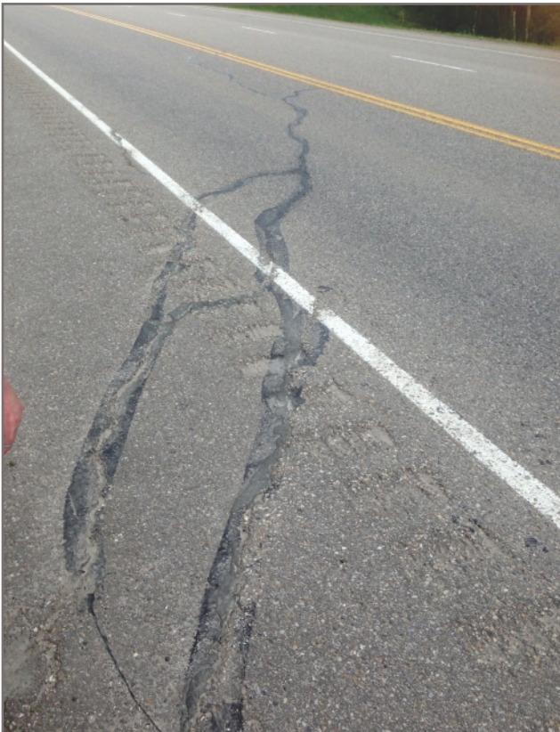
Photo 6: Pavement cracking at west flank of slide sealed in 2010
