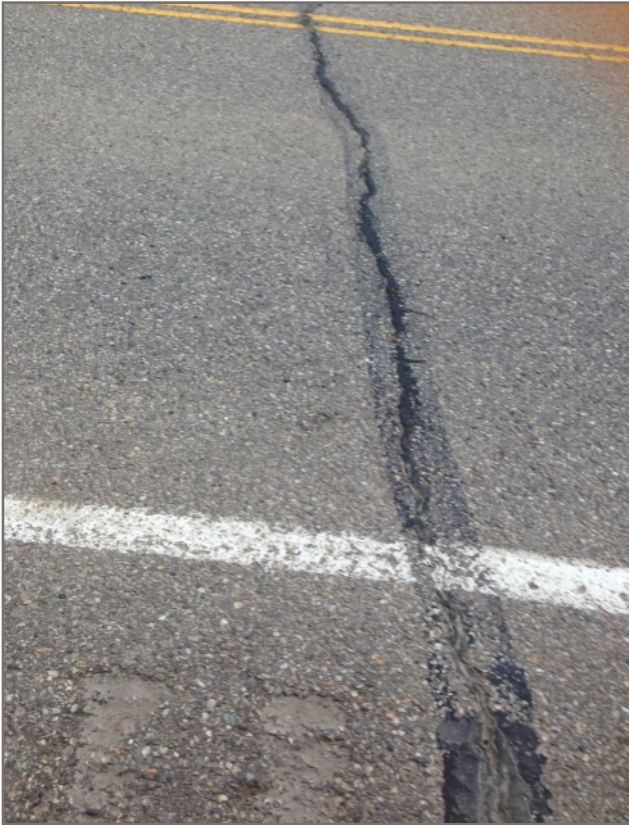
Photo 1: Pavement cracking at east flank of the slide area sealed in 2010
