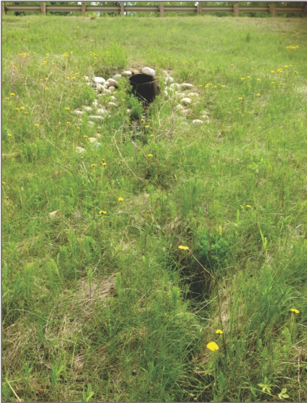
Photo 3: Sparse riprap armoring at east culvert outlet
