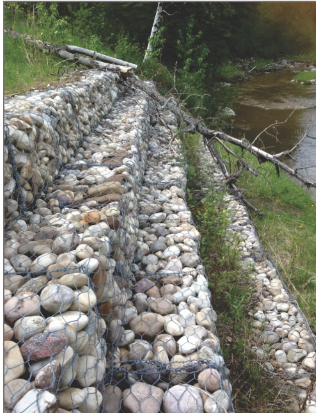
Photo 7: Modeste Creek at toe of sideslope protected from erosion with Gabion baskets
