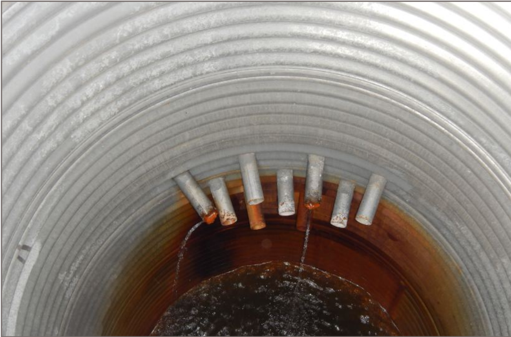
Photo 3: West drainage gallery - two of nine drains in operation
