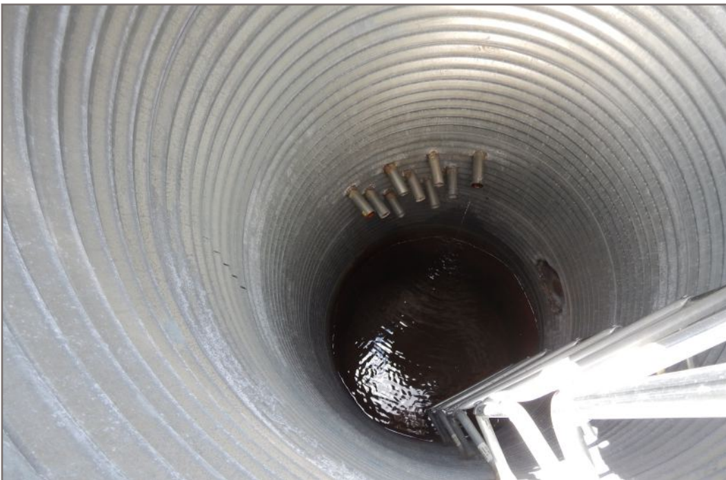
Photo 2: East drainage gallery - one of nine drains in operation
