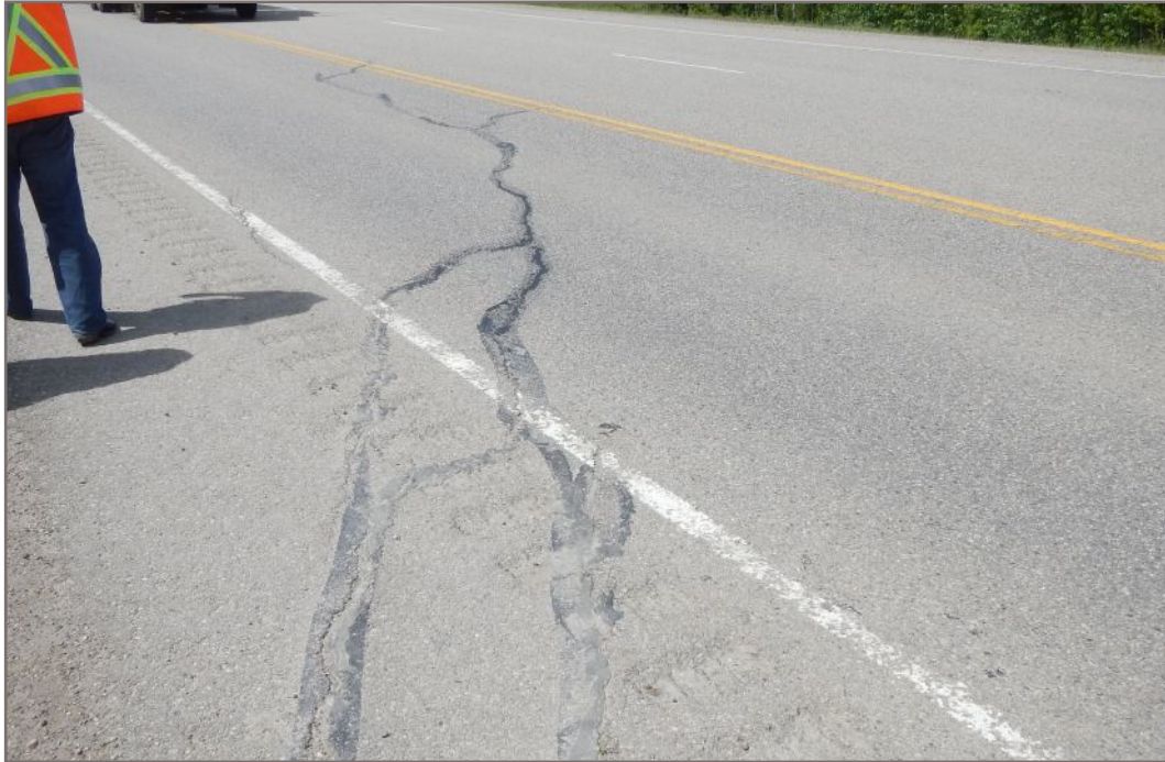
Photo 5: Pavement cracking near west flank of slide sealed in 2010.
