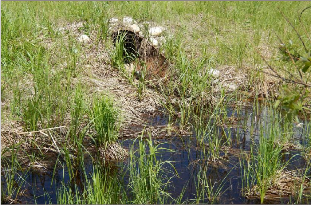
Photo 1: Inlet of east culvert above base of ditch leading to ponding
