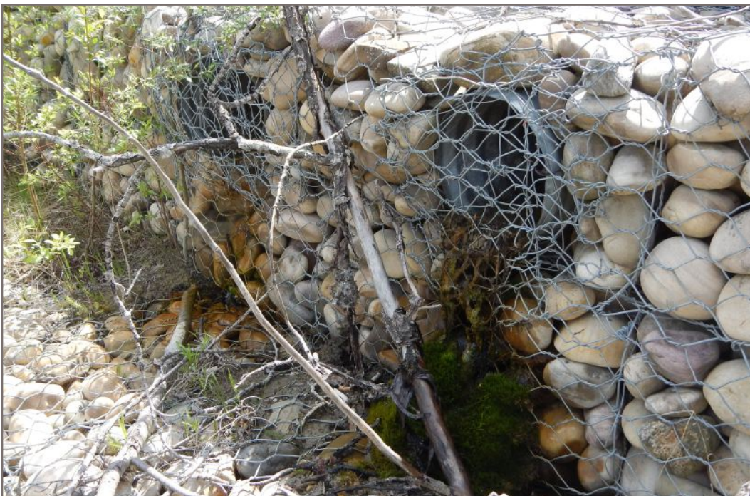
Photo 4: Gabion basket wall located at toe of sideslope adjacent to Modeste Creek. Culvert conveying groundwater from drainage galleries to Modeste Creek.
