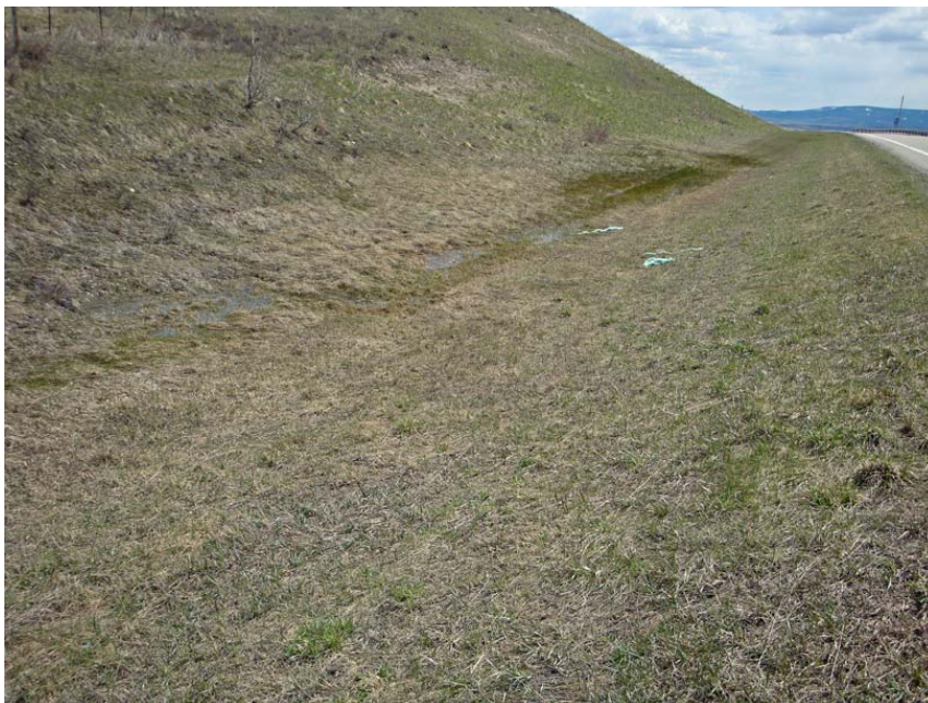
Photo S43-4 (May 2014) Standing in the upslope ditch looking towards the southeast up the ditch invert. The area is relatively flat and had ponded water.
