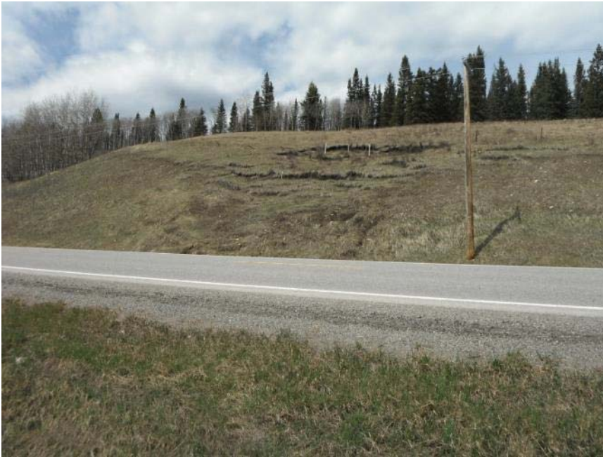
Photo S45-5 (May 2014) – Standing at the West Site looking towards the northeast at the backslope sliding.
