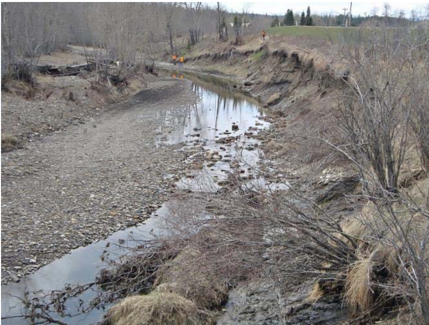
Photo S45-2 (May 2014) – Standing at the creek bank at the east end of the East Site, looking towards the southwest at the bank erosion. Similar location as Photo 1, note the low flow and relatively unchanged bank conditions relative to the 2013 conditions.
