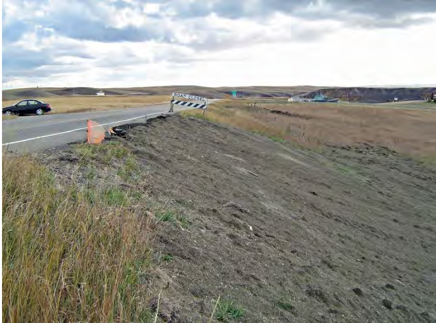
Photo S46-1 (2007) At the North Site on the west side of the road embankment looking towards the south at the area where landslide damage had occurred and recently been regraded.
