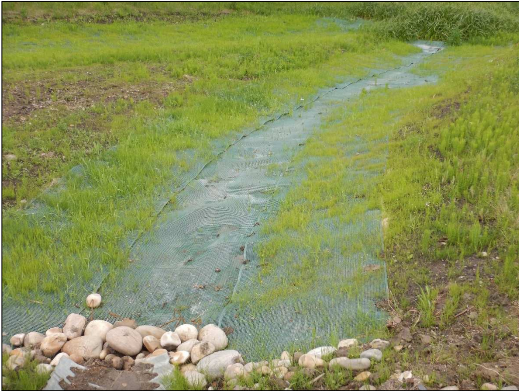
Photo 6: Erosion and sediment control installed along drainage path immediately west of the site
