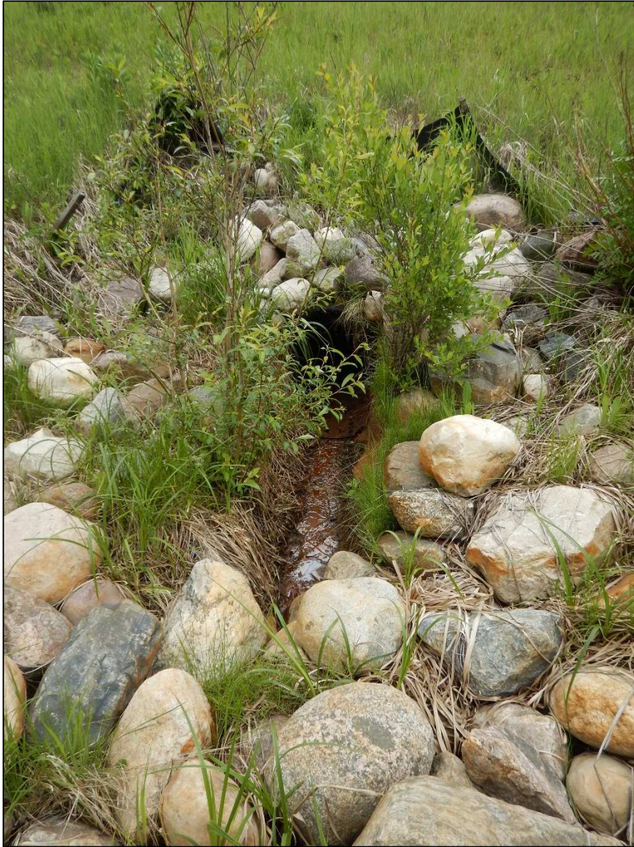
Photo 7: West culvert inlet protection well vegetated
