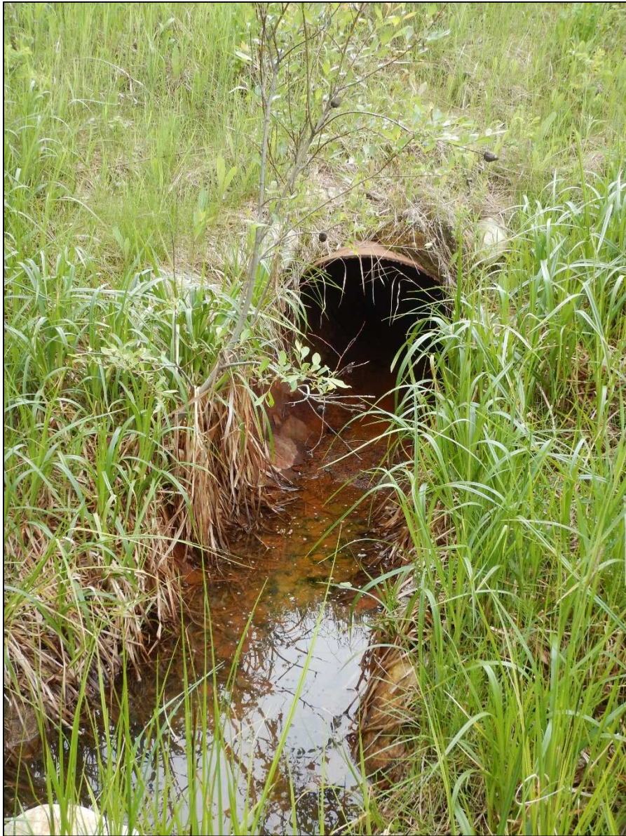
Photo 5: Ponding water at west culvert outlet
