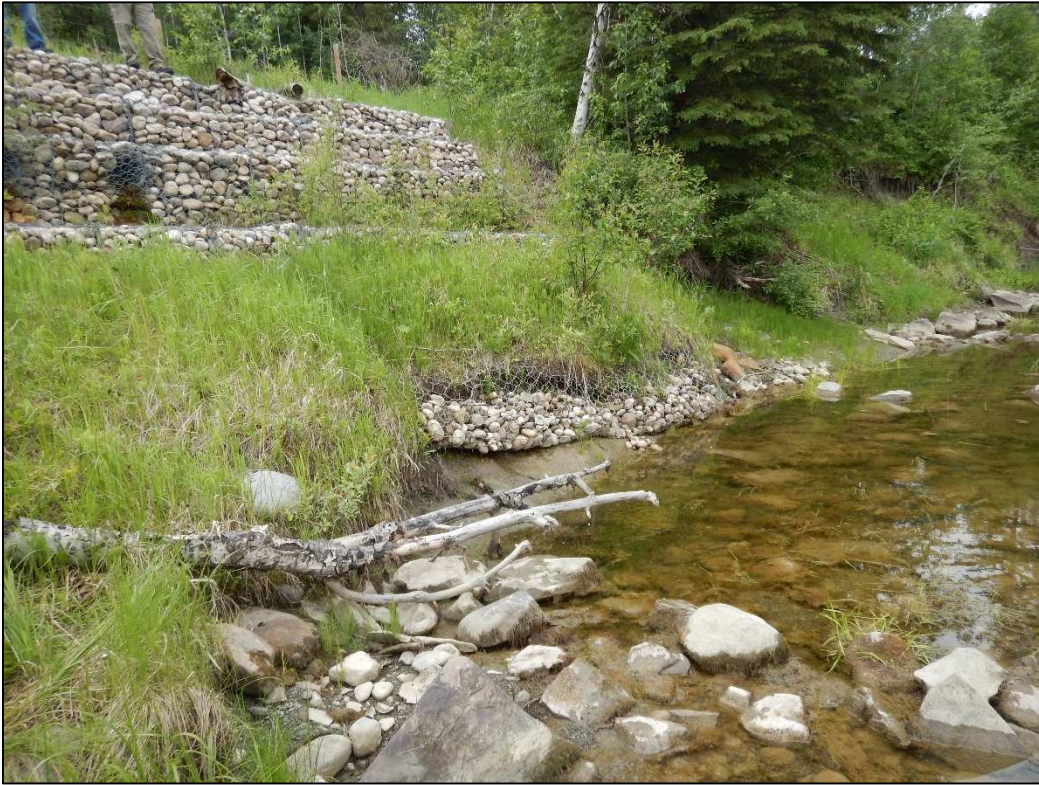
Photo 4: Erosion and deformation of gabion baskets along riverbank at toe of slope
