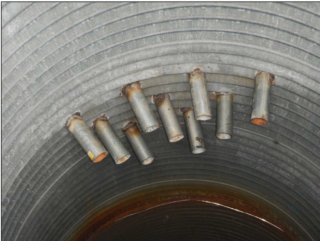
Photo 3: East drainage gallery – zero of nine running
