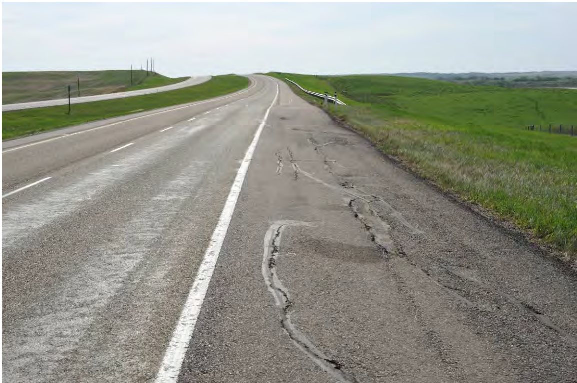
Photo 1 Site Conditions May 19, 2010
