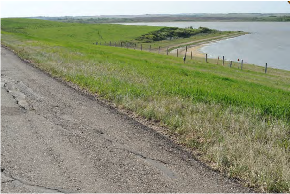
Photo 2 Site Conditions May 19, 2010
