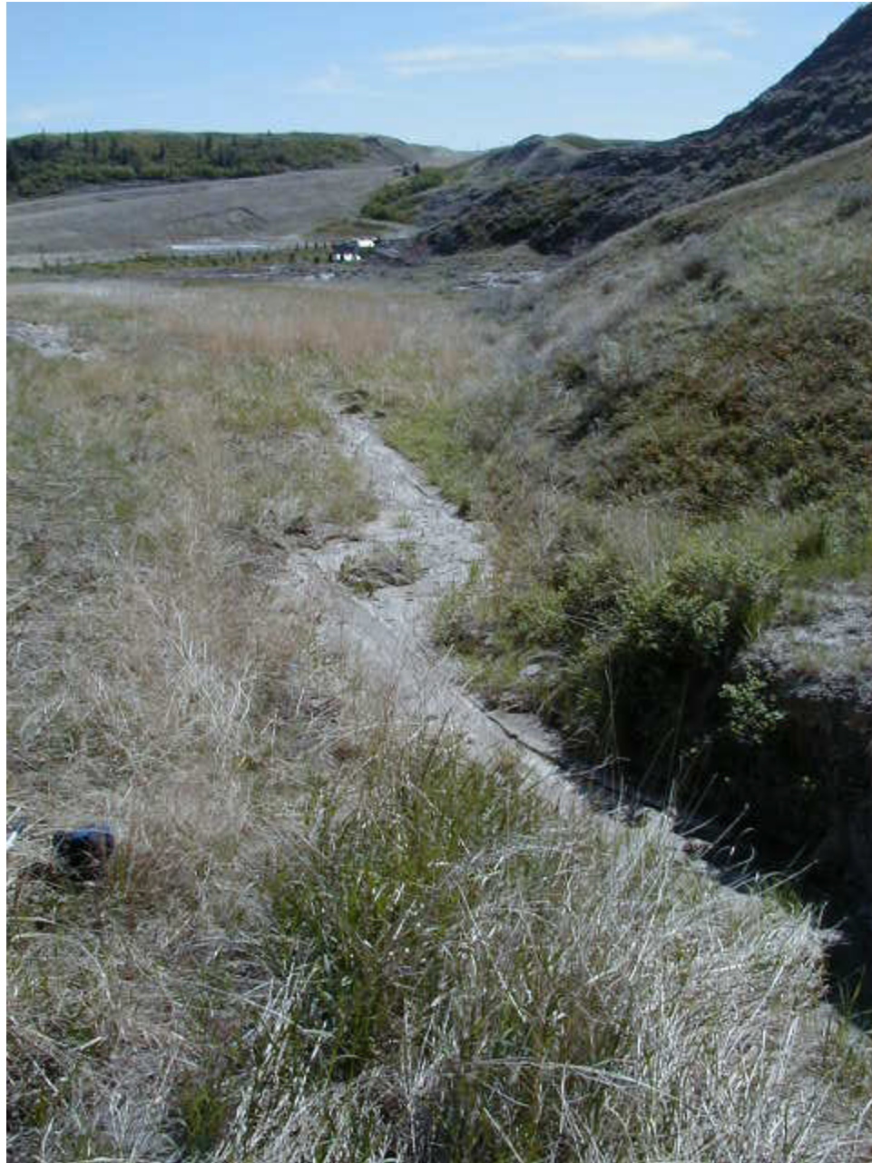
South end of erosion gully
