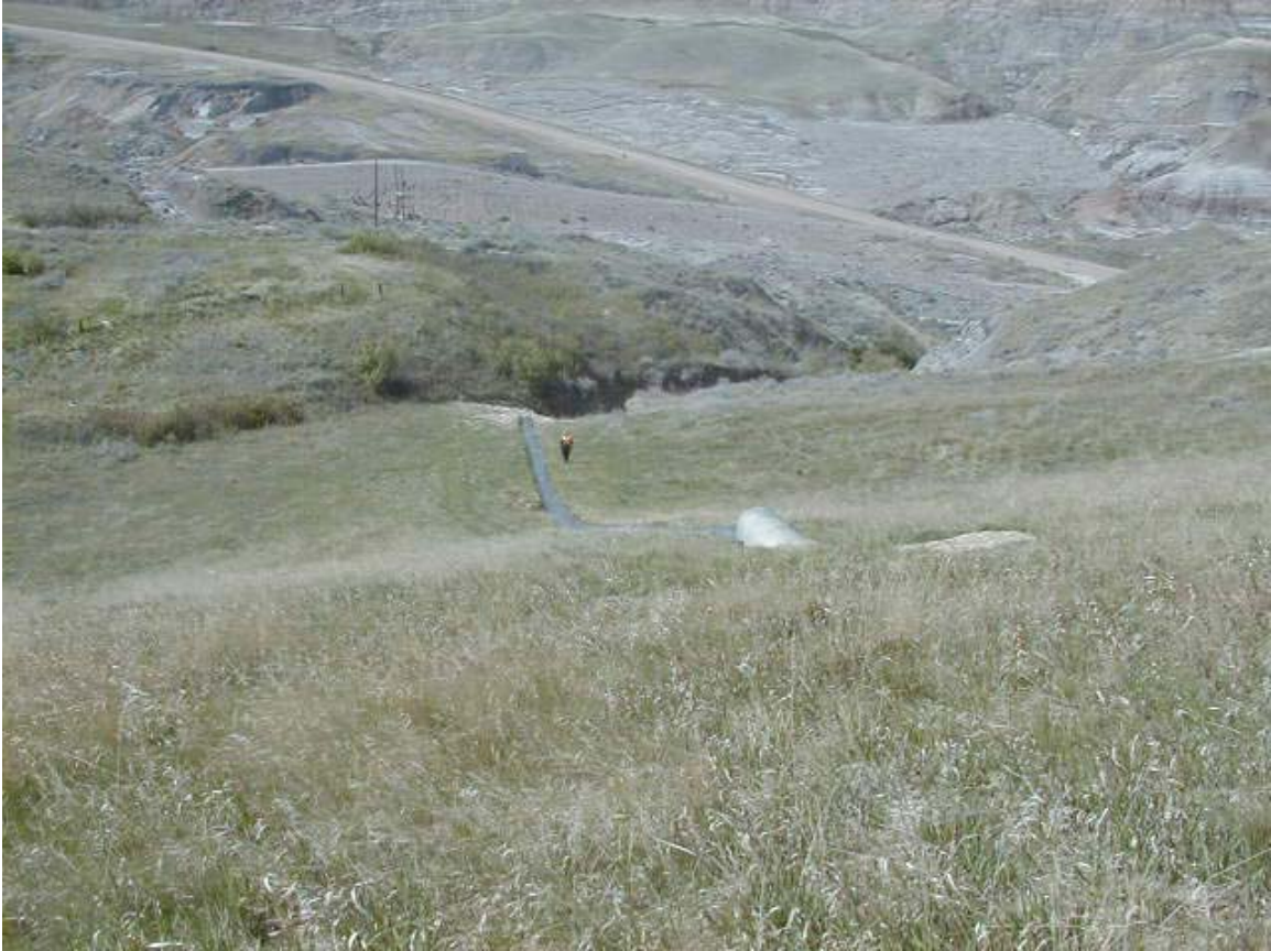
Outlet of lower culvert
