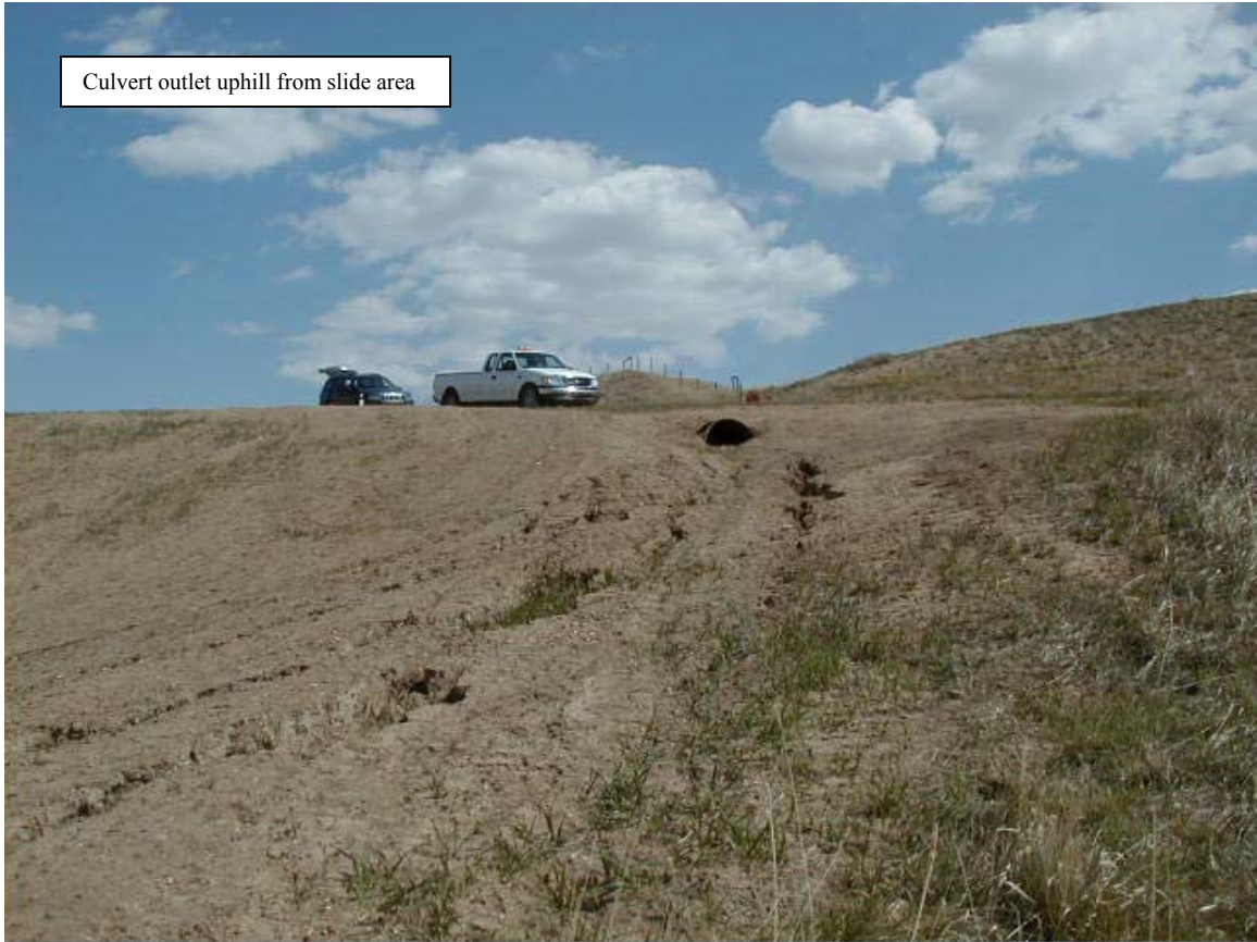
Erosion downstream of outlet
