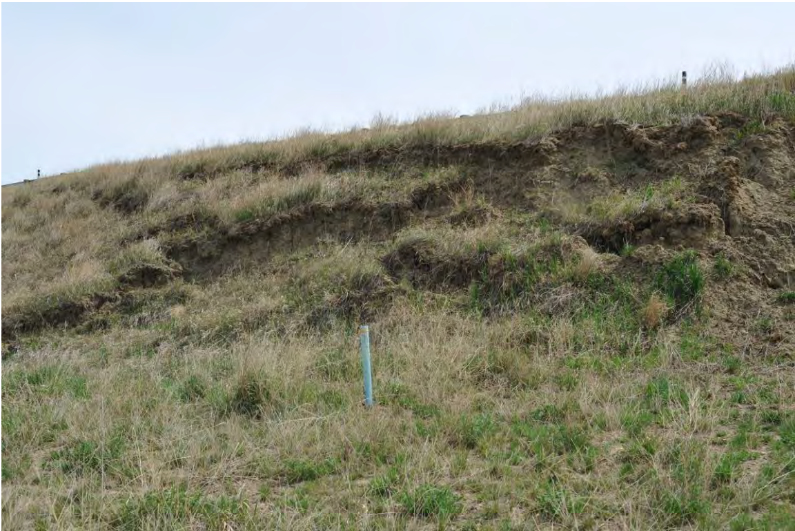
Photo 1 Site Conditions May 18, 2010 (SI4 in foreground, see Figure 1)
