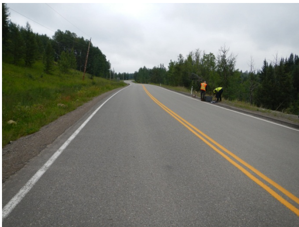
No cracking, settlement or other signs of movement in the highway or gravel slope observed
