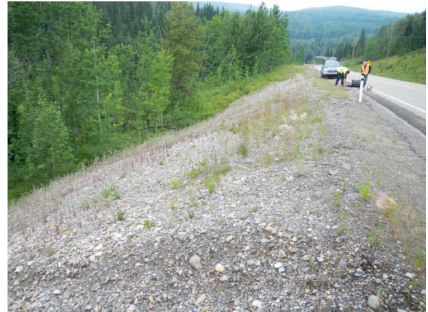
No cracking, settlement or other signs of movement in the highway or gravel slope observed
