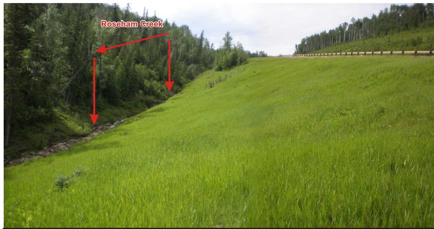
Photo 2 Looking south upgrade (towards Grande Cache) along mid-height of Cutbank River valley slope - About 400m of sidehill alignment (approach to Cutbank River) runs parallel to Rosebud Creek (tributary to Cutbank River) - Rosebud Creek is a straight channel and downcutting along a steep (7%) gradeline - Slumping of creek banks along Rosebud Creek at toe of highway sideslope (see photo #13 to 14 for bank slumping movements) deteriorating and starting to destabilize effect on this sidehill highway alignment. (See photos# 8, 11 to 13 for development of tension cracks)
