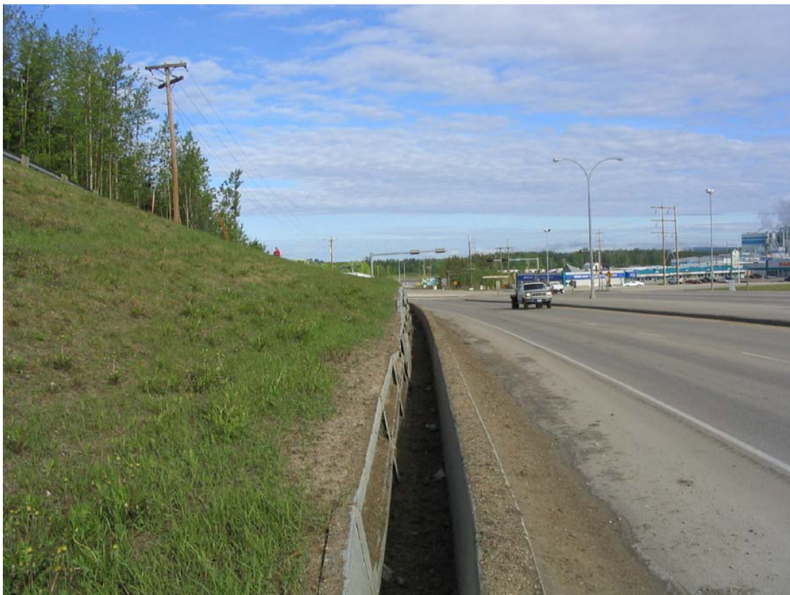
PHOTO 12 BIN WALL, STATION 1+200 LOOKING WEST
