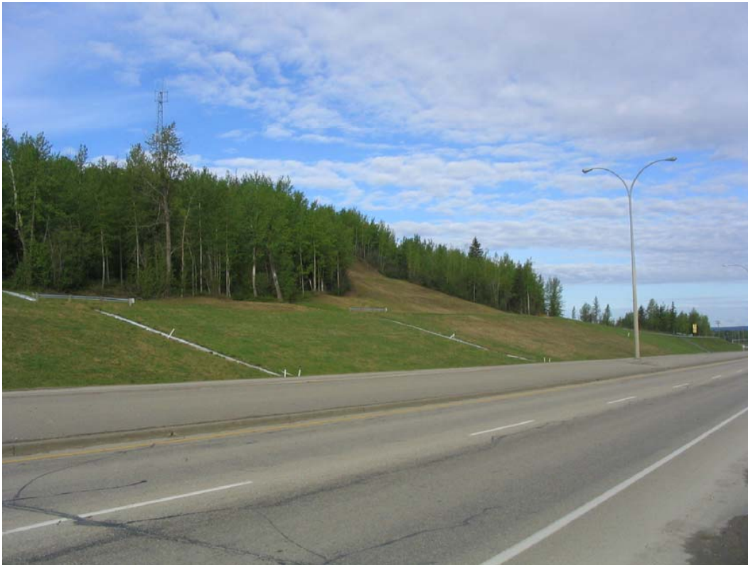
PHOTO 8 AREA OF PREVIOUS BACKSLOPE REPAIR (LOOKING SOUTHWEST)
