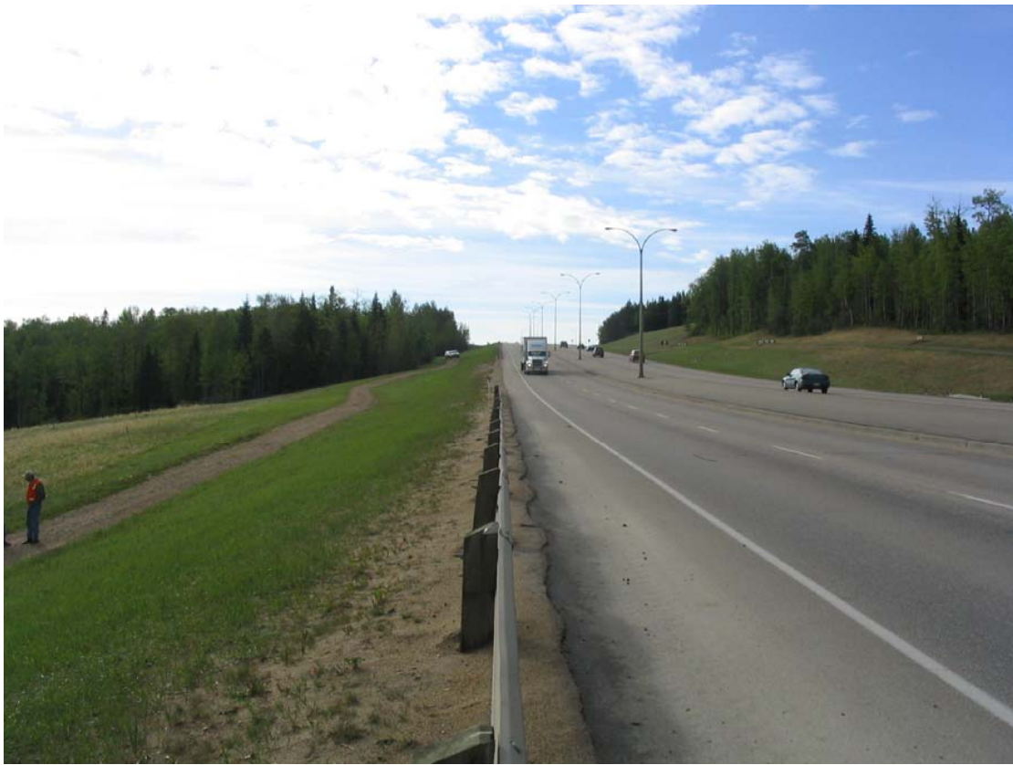
PHOTO 5 LOOKING EAST ALONG NORTH GUARDRAIL
