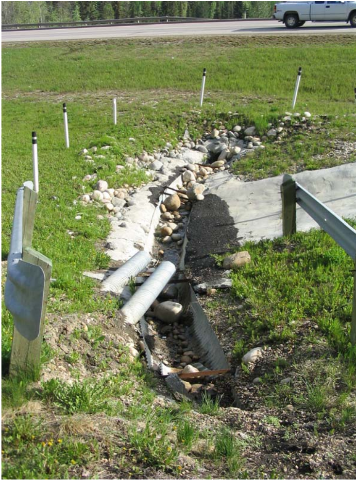
PHOTO 7 SUBDRAIN AND CULVERT OUTLETS NEAR STATION 1+680 (SOUTH OF HIGHWAY)
