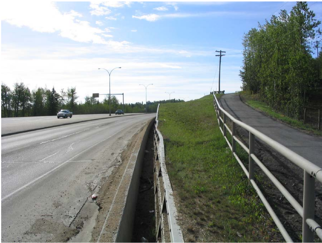
PHOTO 11 BIN WALL, STATION 1+200 LOOKING NORTHEAST
