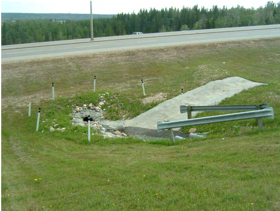
Photo 5 – Subdrains and culvert outlet near Sta. 1+680, June 5, 2006
