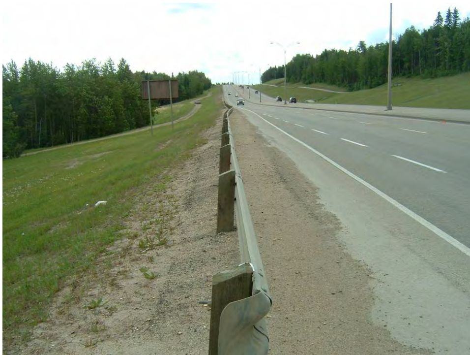
Photo 4 – Looking east along north guardrail (west of Photo 3), June 5, 2006
