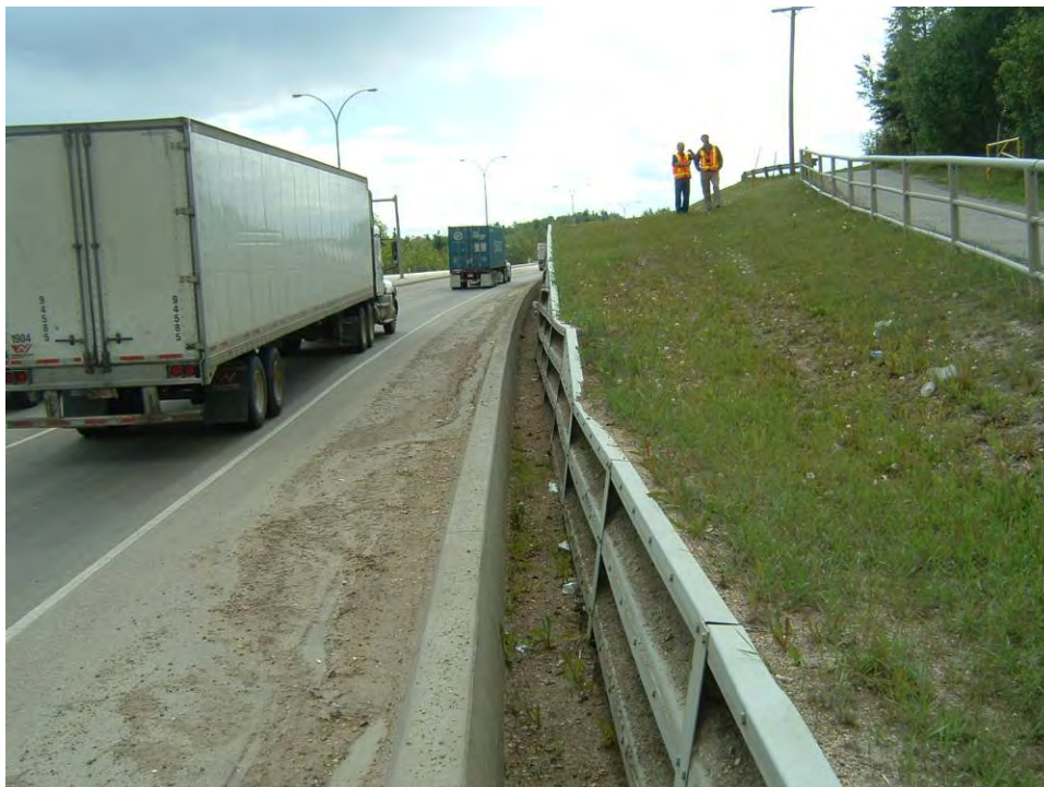
Photo 10 – Looking east at bin wall (Sta. 1+200), June 5, 2006
