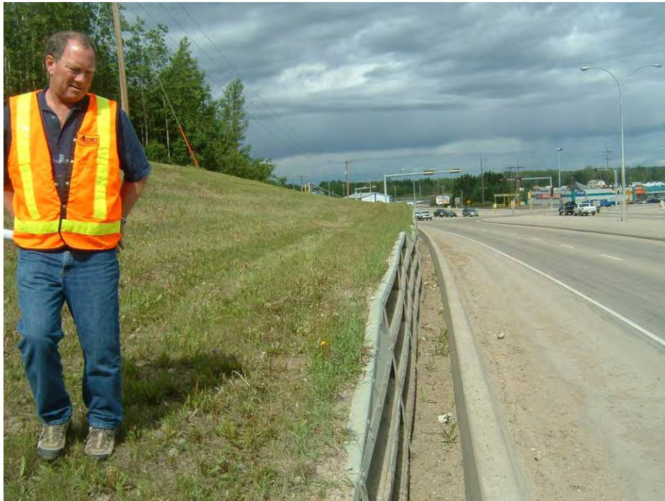
Photo 9 – Looking west at bin wall (Sta. 1+200), June 5, 2006
