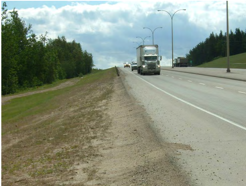
Photo 3 – Looking east along north guardrail, June 5, 2006
