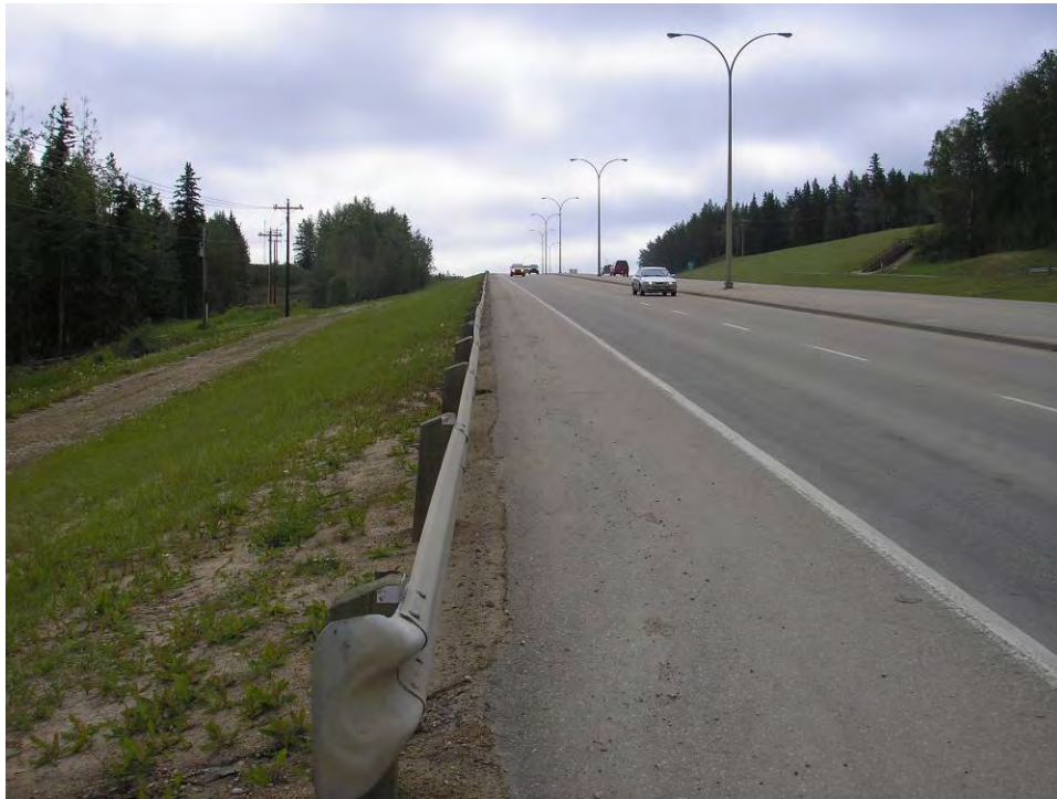
Photo 3 – Looking east along north guardrail, June 11, 2007.
