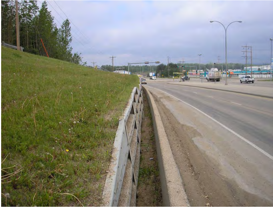
Photo 9 – Looking west at bin wall (Sta. 1+200), June 11, 2007.
