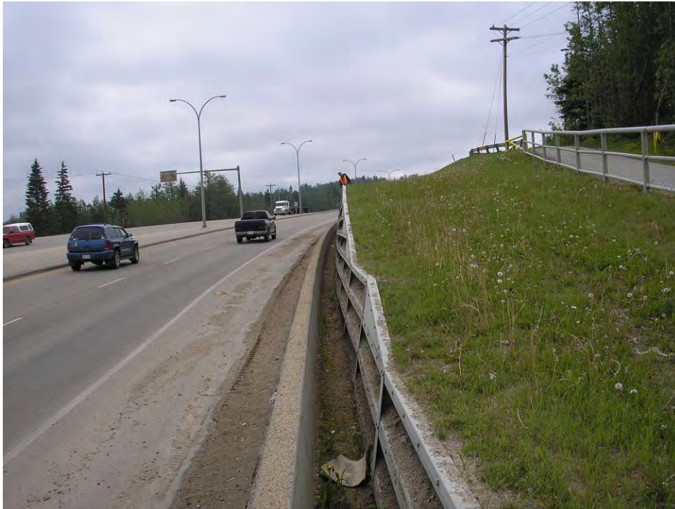
Photo 10 – Looking east at bin wall (Sta. 1+200), June 11, 2007.
