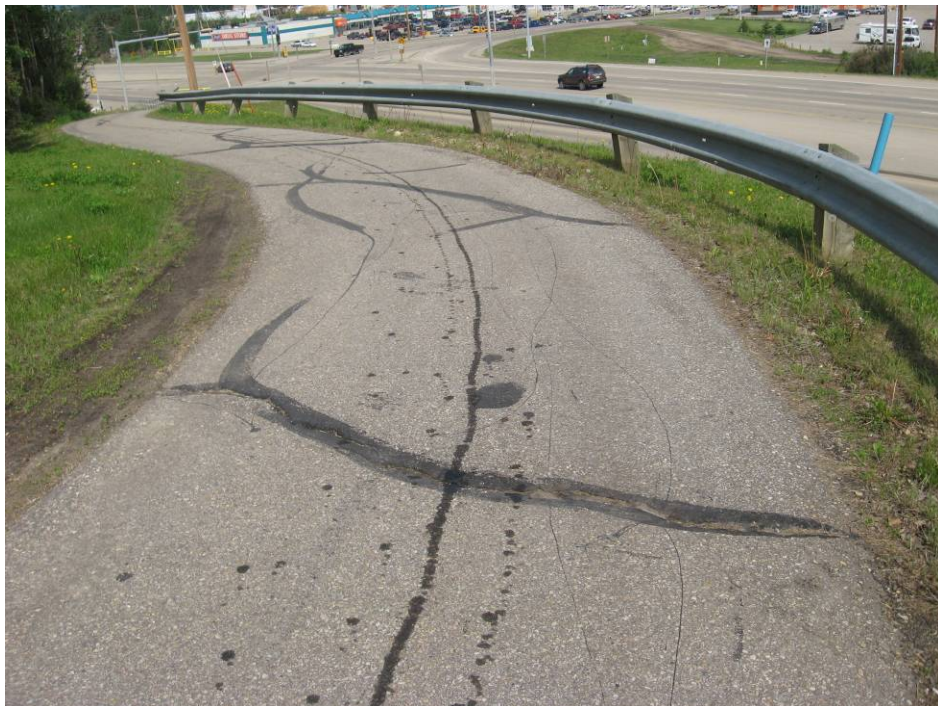
Photo 6 – Looking west at cracks above bin wall, June 11, 2008.
