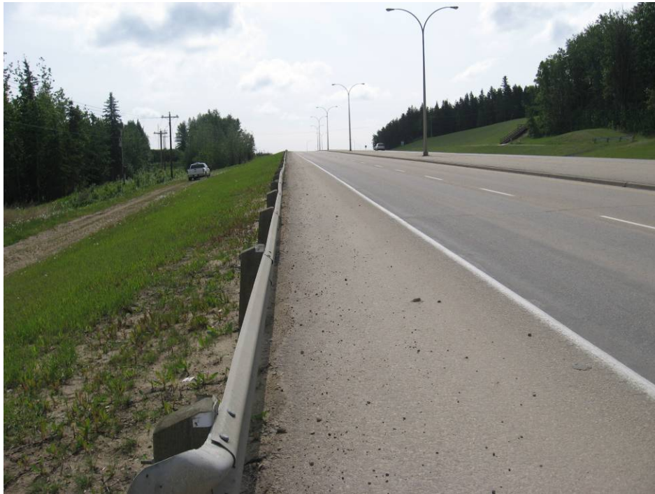
Photo 3 – Looking east along north guardrail, June 11, 2008.
