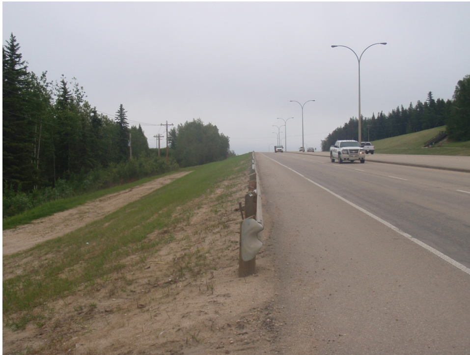
Photo 5 – Looking east along north guardrail (June 15, 2010).
