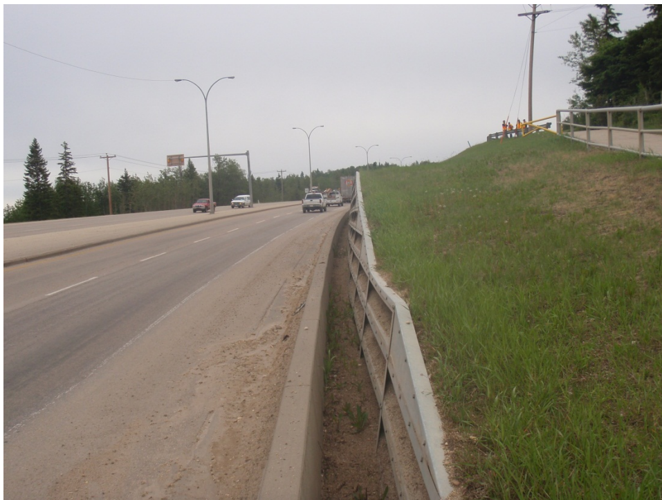
Photo 12 – Looking east at bin wall (Station 1+200) (June 15, 2010).
