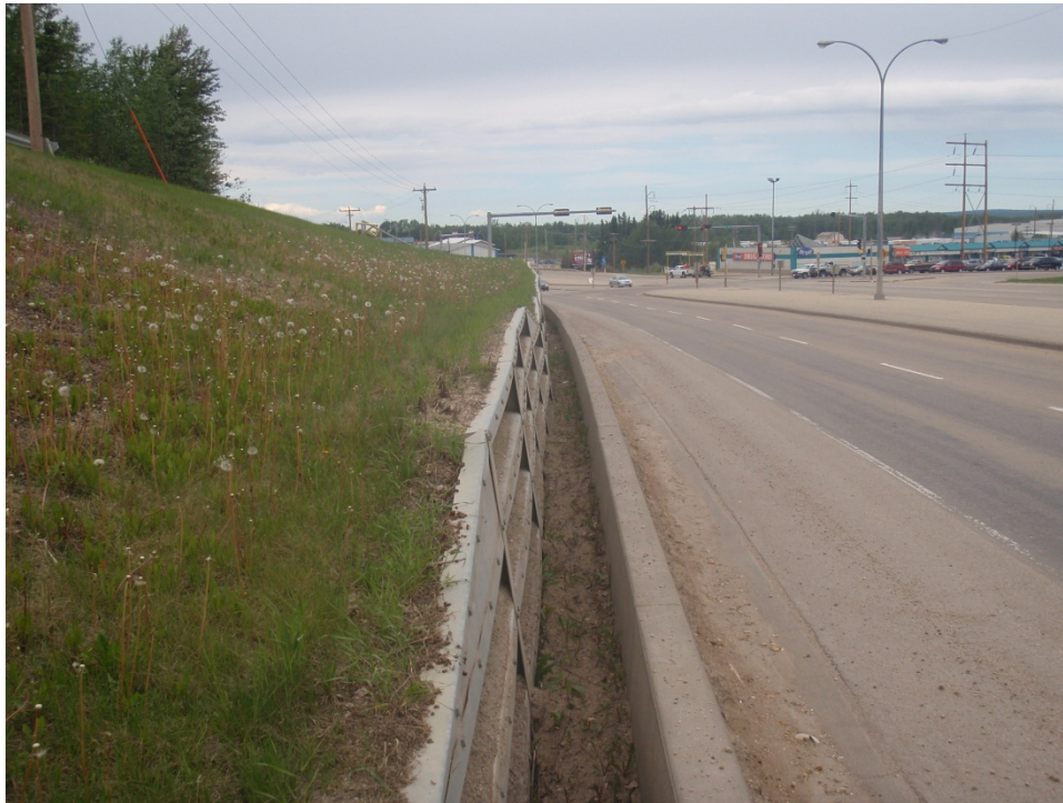
Photo 11 – Looking west at bin wall (Station 1+200) (June 15, 2010).
