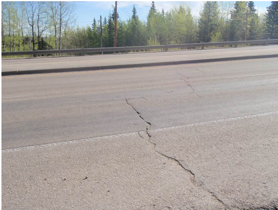
Photo 6 – Looking northeast at culvert dip at Station 1+850 (May 17, 2011).
