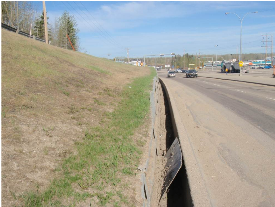
Photo 9 – Looking west at bin wall (Station 1+200) (May 17, 2011).
