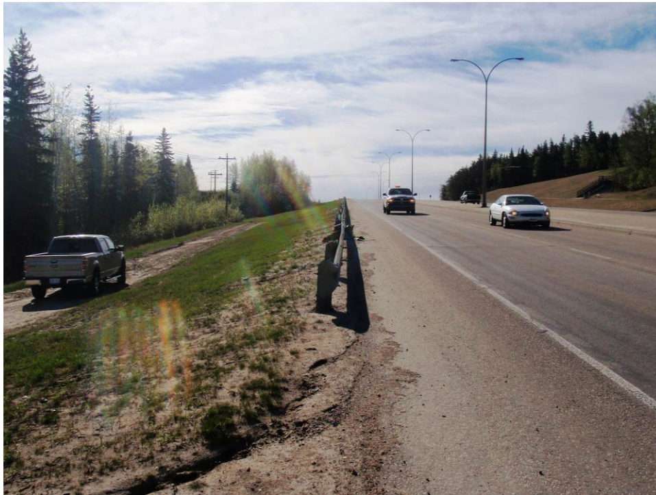
Photo 5 – Looking east along north guardrail (May 17, 2011).
