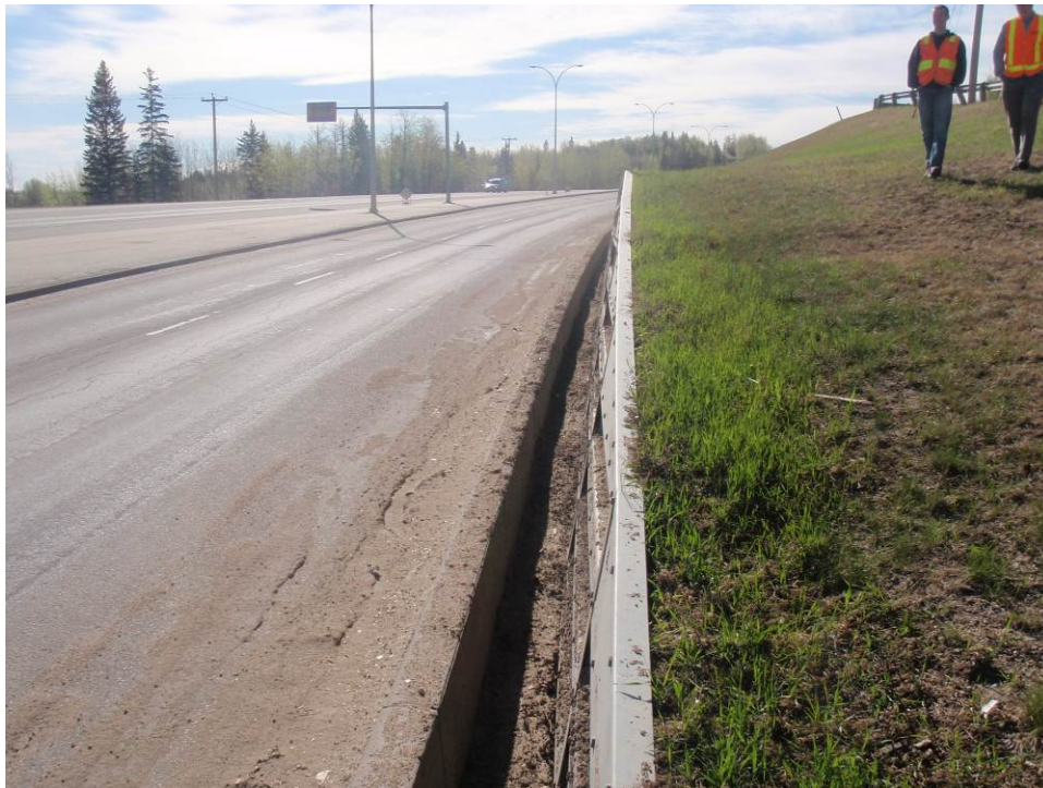
Photo 10 – Looking east at bin wall (Station 1+200) (May 17, 2011).
