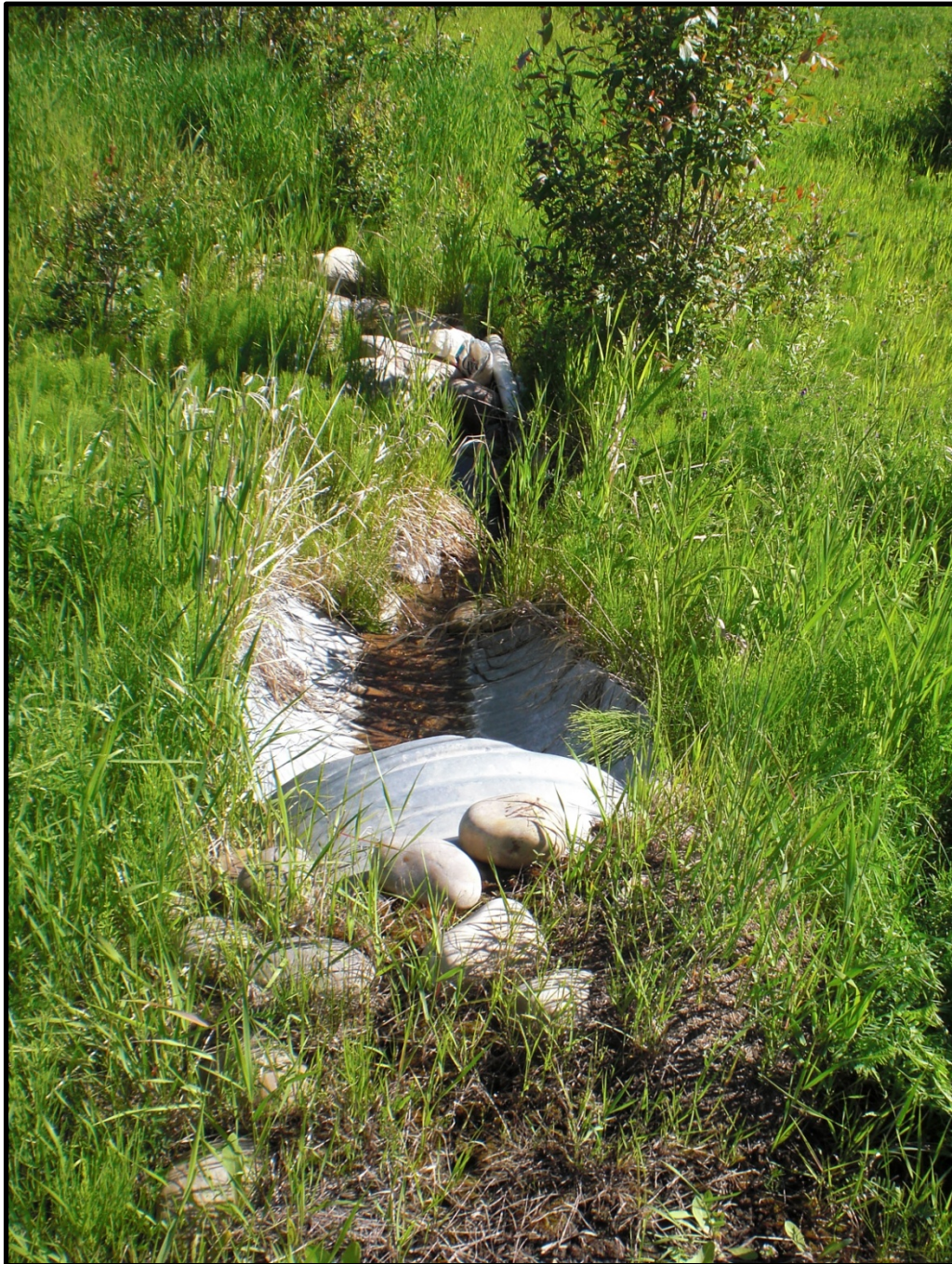
PHOTO 10: Culvert outlet at approximately 1+650.
