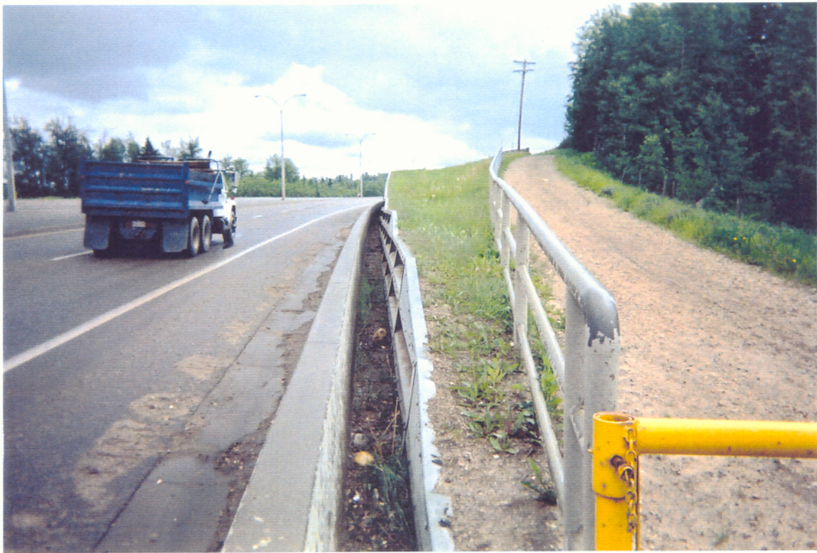
BIN WALL, STATION 1+200 LOOKING NORTHEAST
