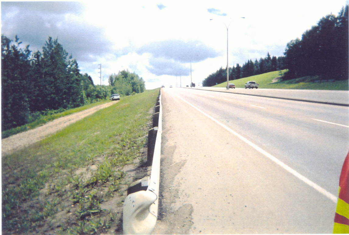
LOOKING EAST AT UPPER GUARDRAIL
