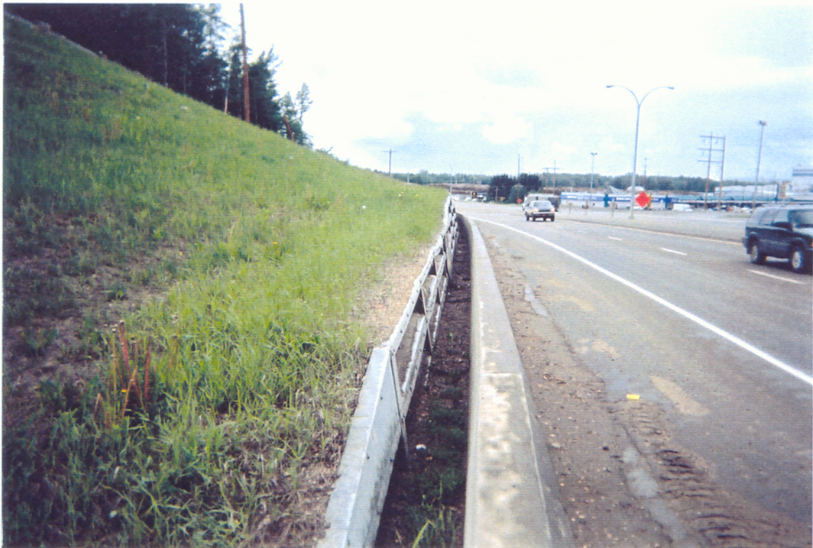
BIN WALL, STATION 1+200 LOOKING WEST
