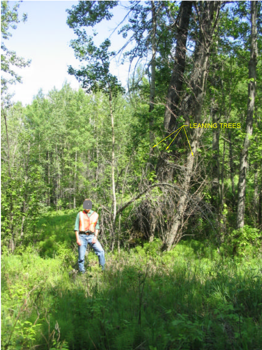
PHOTO 3 LOOKING WEST AT POTENTIALLY UNSTABLE AREA DOWNSLOPE OF THE ROADWAY
