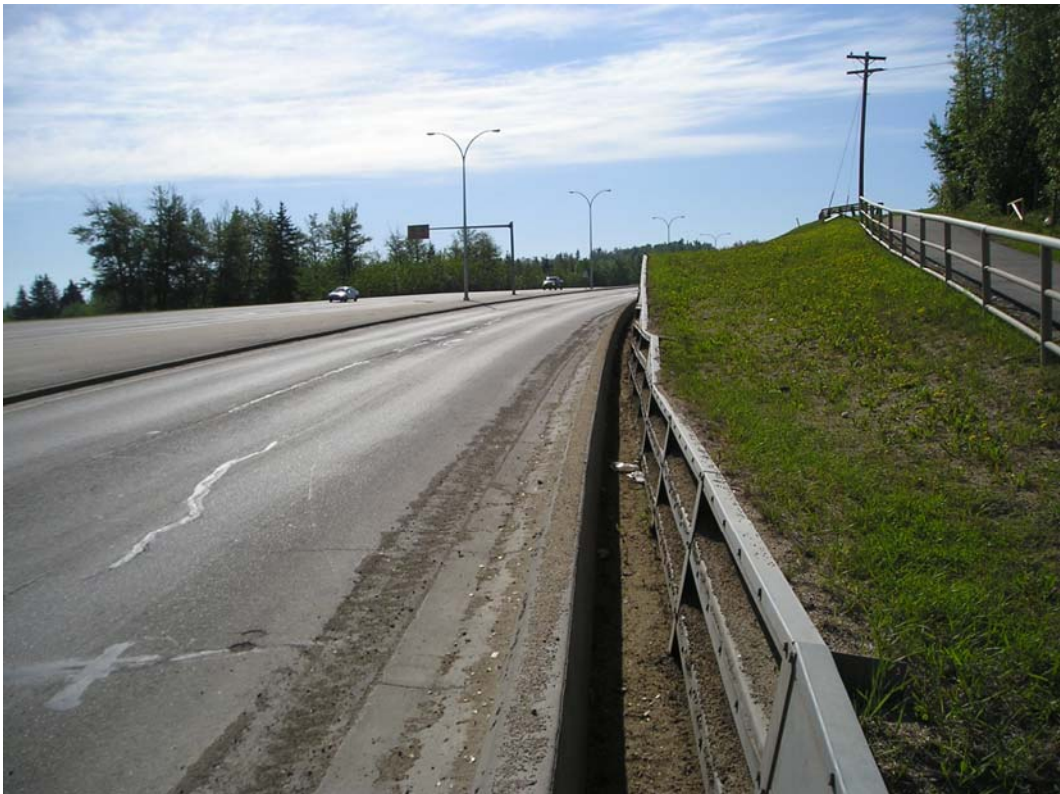
Photo 10 – Bin wall Station 1+200 looking northeast.
