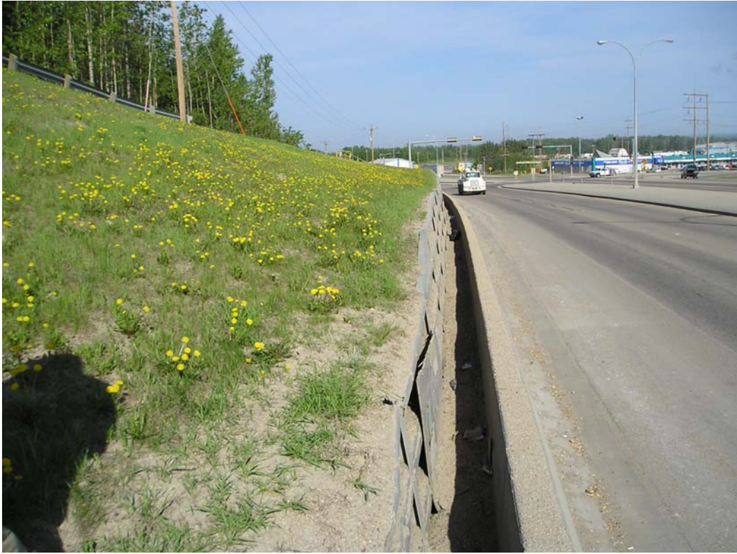
Photo 9 – Bin wall Station 1+200 looking west.
