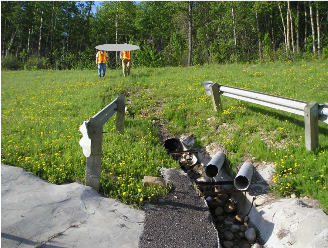
Photo 5 – Subdrains and culvert outlet near Station 1+680 (south of highway).
