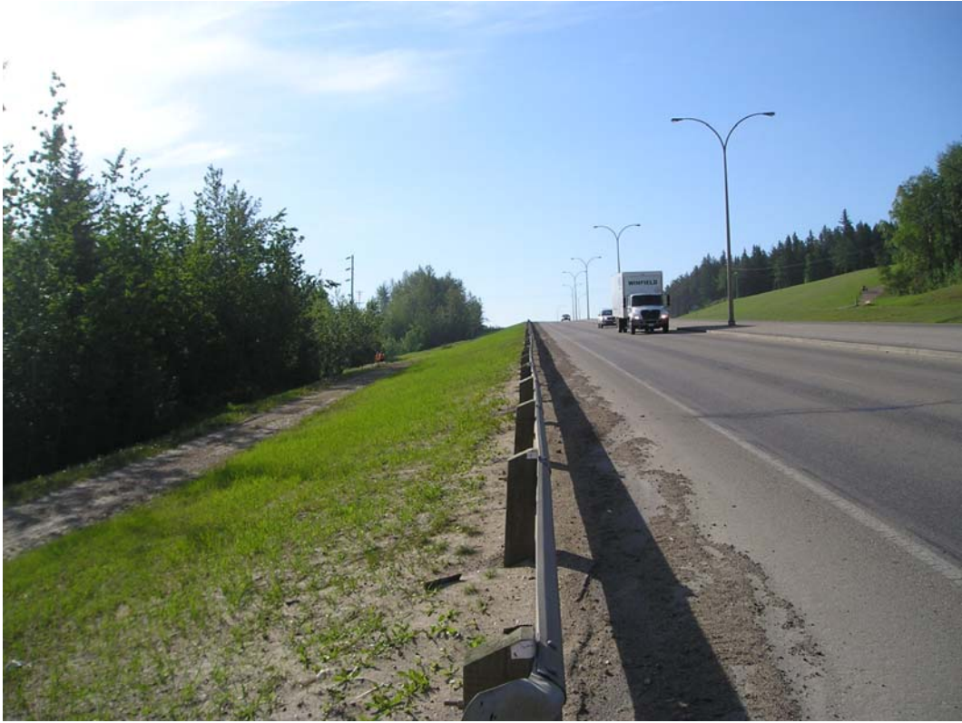
Photo 3 - Looking east along north guardrail.
