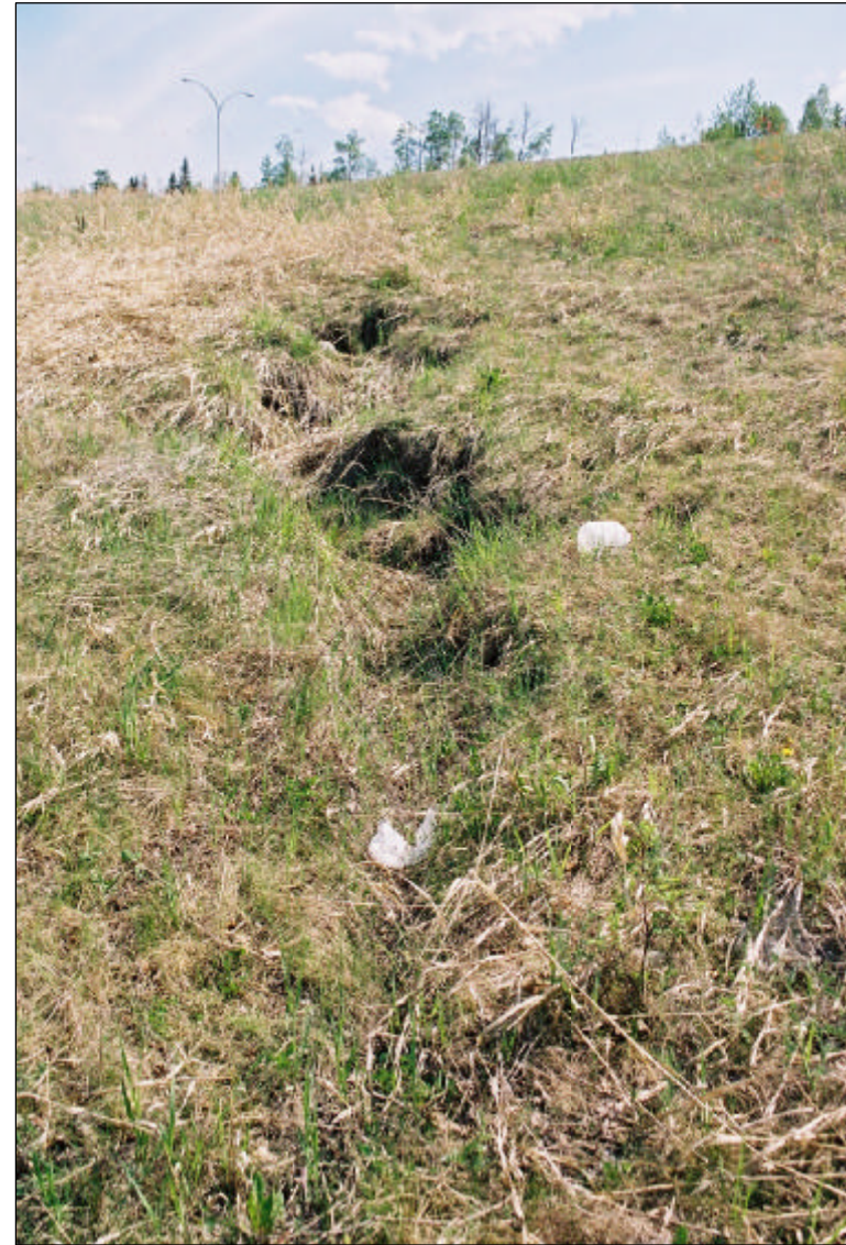
EROSION GULLY WEST OF TOE BERM
