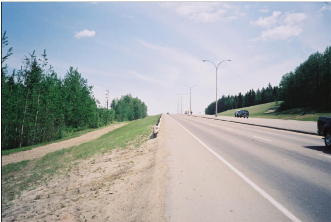
LOOKING EAST AT UPPER GUARDRAIL
