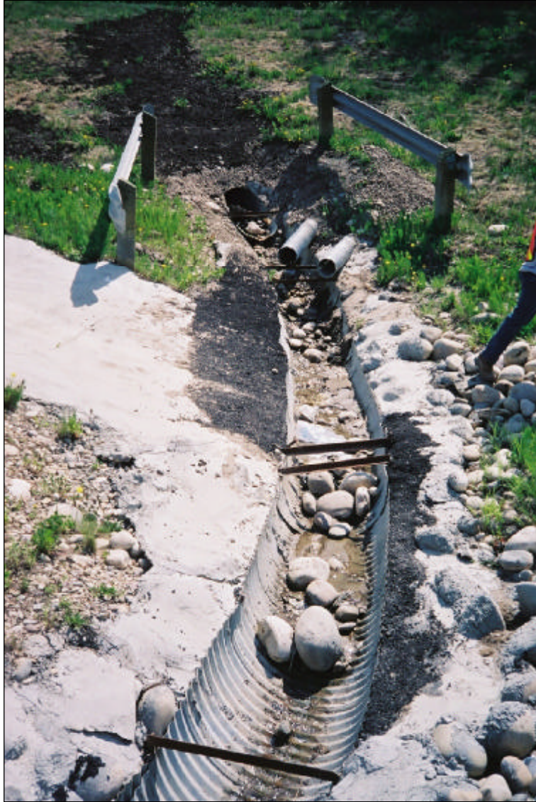
SUBDRAIN AND CULVERT OUTLETS NEAR STATION 1+680 (SOUTH OF HIGHWAY)
