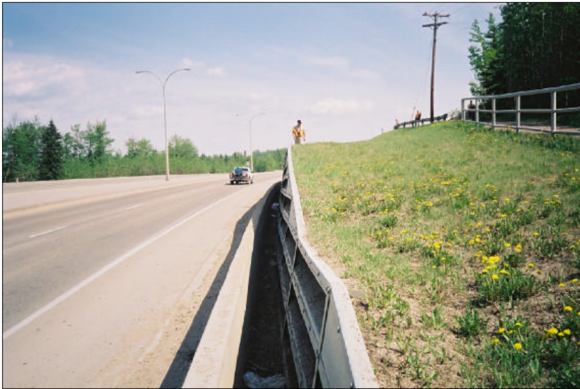
BIN WALL, STATION 1+200 LOOKING NORTHEAST
