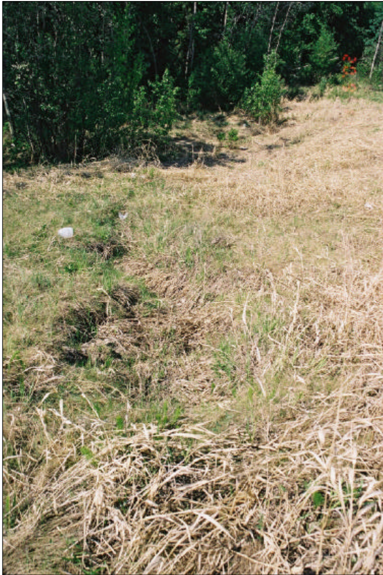
EROSION GULLY WEST OF TOE BERM
