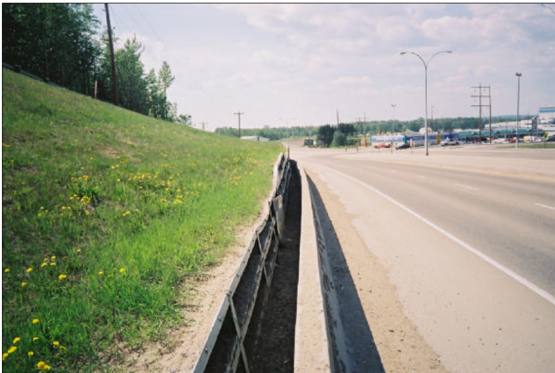
BIN WALL, STATION 1+200 LOOKING WEST
