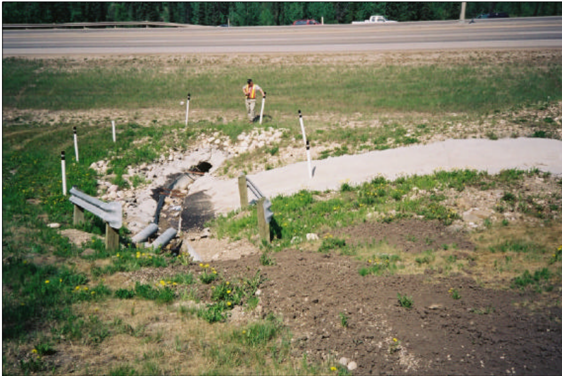
SUBDRAIN AND CULVERT OUTLETS NEAR STATION 1+680 (SOUTH OF HIGHWAY)
