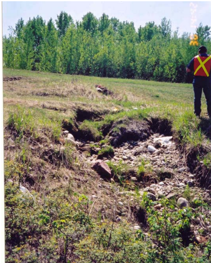
West culvert outlet scour.
