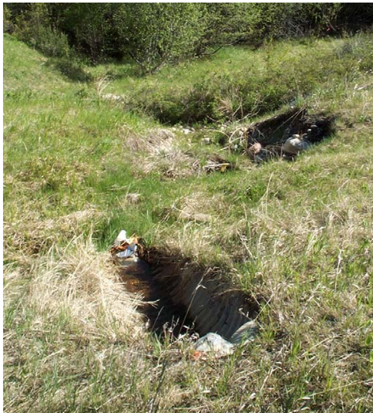
West culvert outlet scour.
