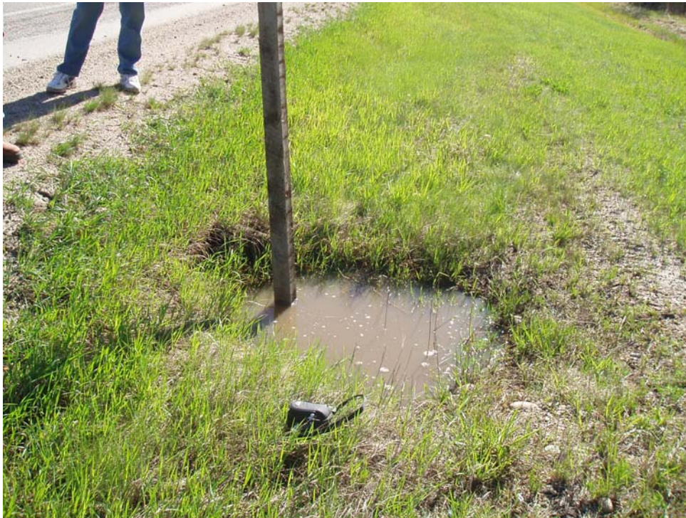
Photo 3 – South side sinkhole (2005).
