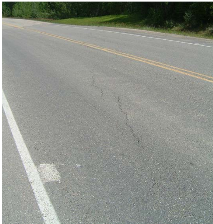
Photo 2 – Pavement cracks (2005).
