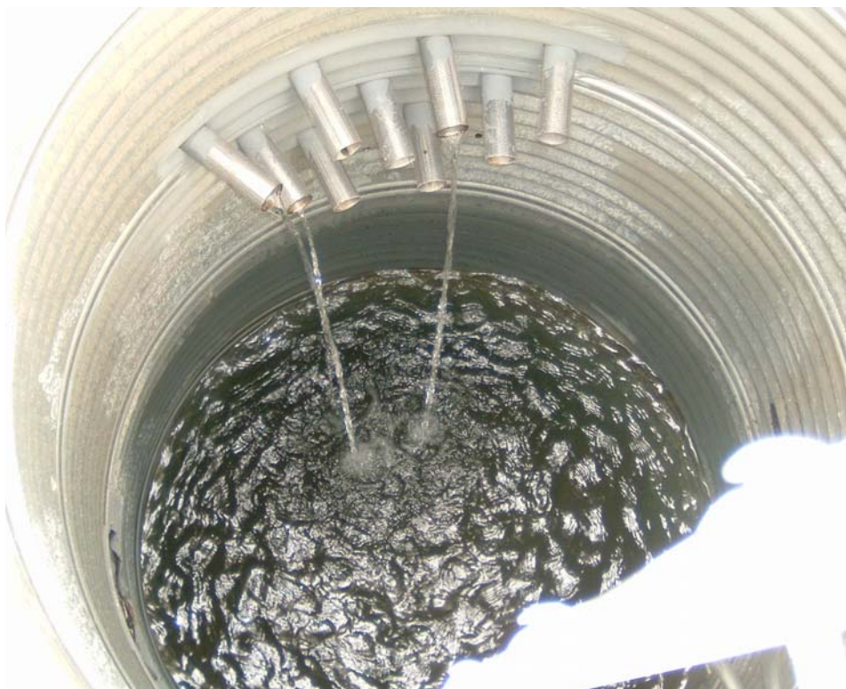
Photo 6 – Subhorizontal drains manhole (photo taken two month after the site visit) (2005).
