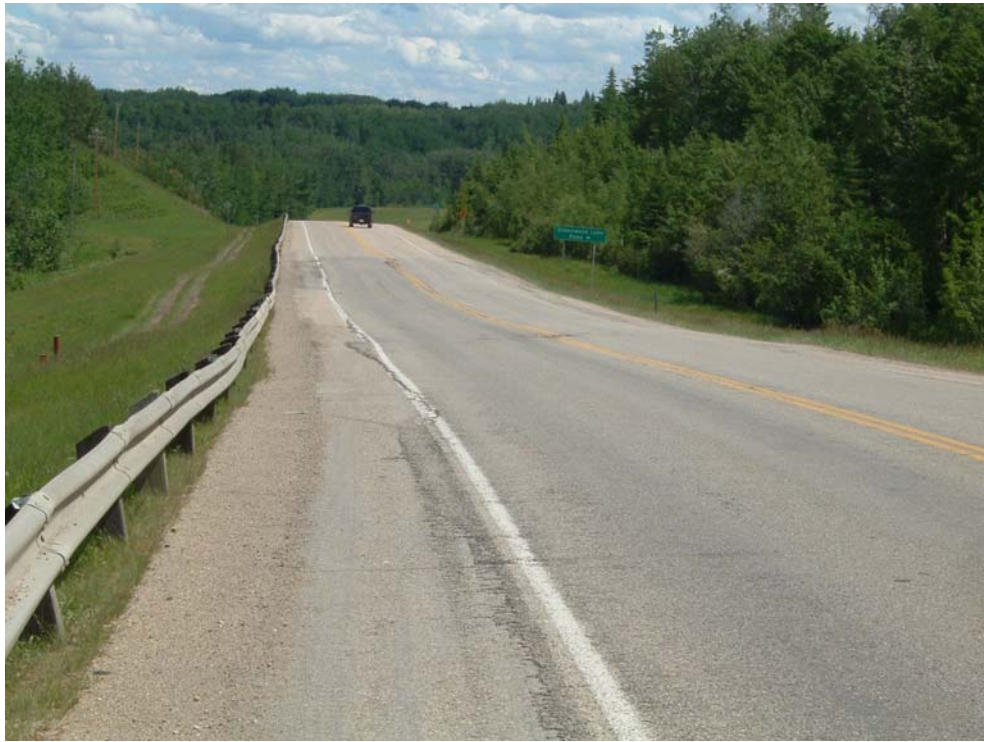
Photo 1. Pavement distress area (looking east), note pavement dips at the centre (2005).
