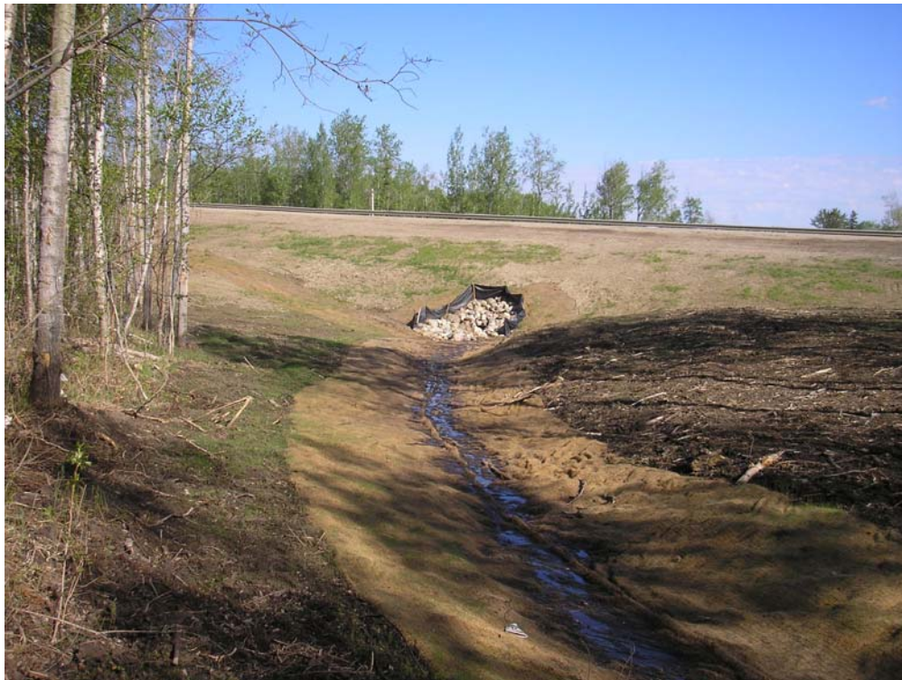
Photo 4 – New culvert inlet and drainage channel (south of highway), May 18, 2006.
