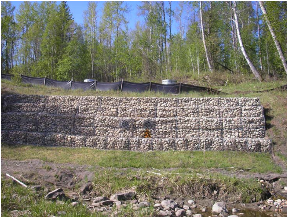
Photo 8 – Gabion outfall structure, May 18, 2006.
