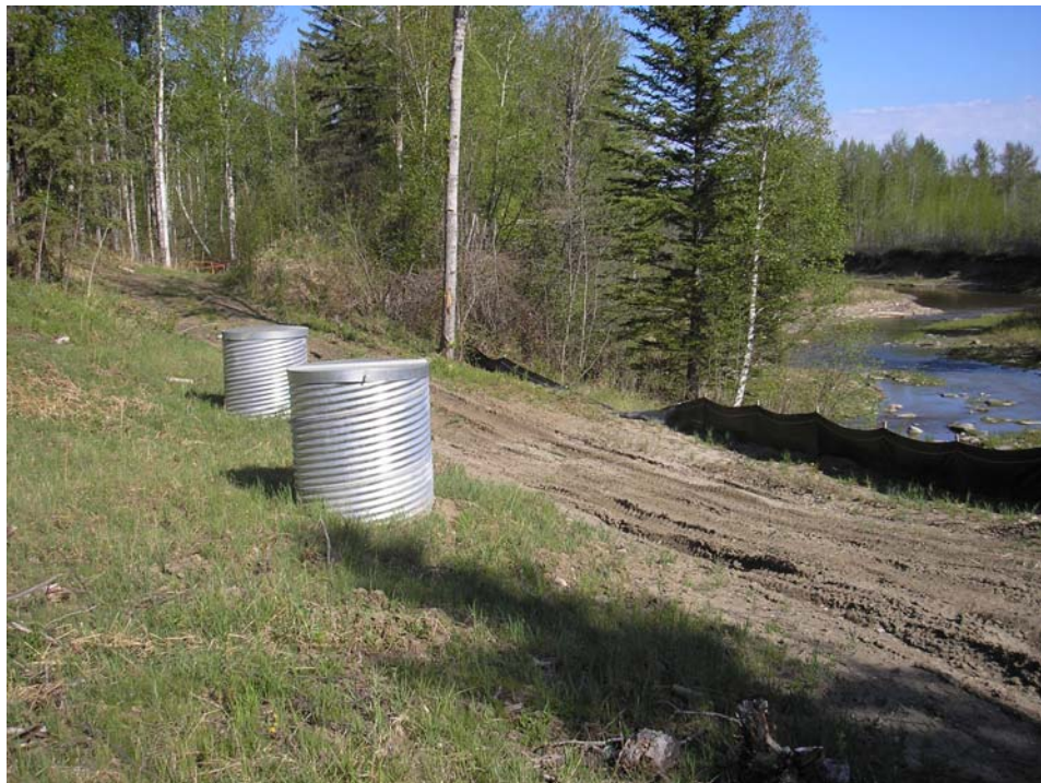
Photo 6 – Subhorizontal drain man access points, (note the knocked down section of the silt fence), May 18, 2006.
