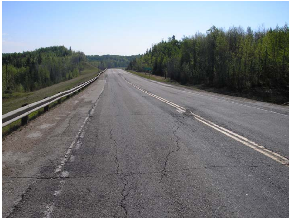
Photo 1. Pavement distress area (looking east), May 18, 2006.
