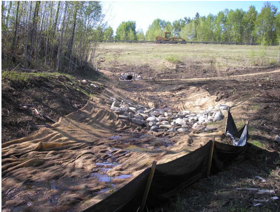
Photo 5 –New culvert outlet and drainage channel (north of highway), May 18, 2006
