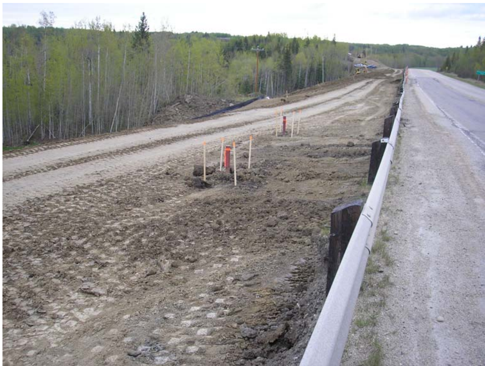
Photo 2 – Climbing lane fill (note the instrumentation being protected).
