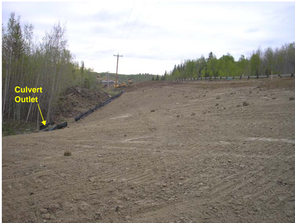
Photo 3 – Sideslope fill oversteepened at the culvert outlet location.
