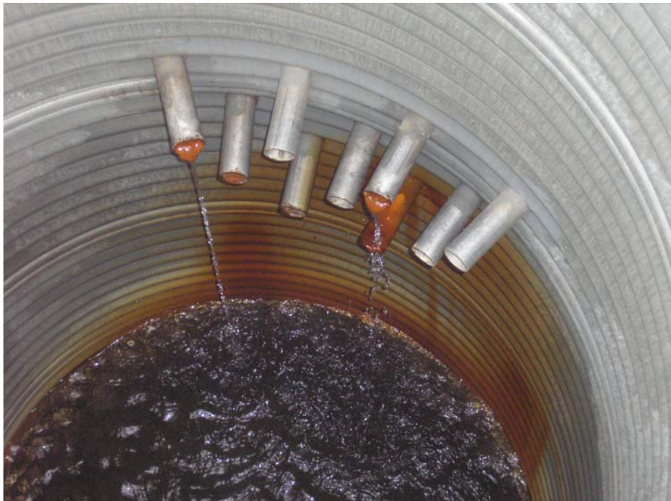
Photo 4 – West collection point subdrains.
