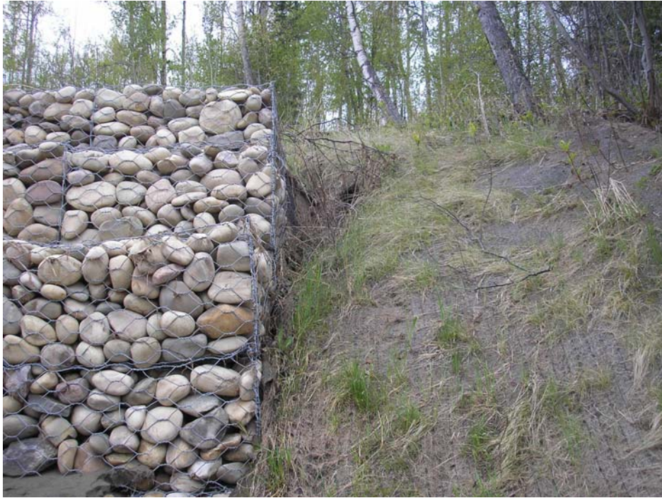
Photo 5 – Gabion wall interface erosion.
