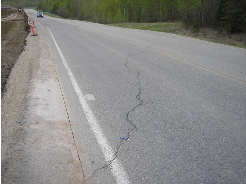
Photo 1 - Pavement distress area (looking east).
