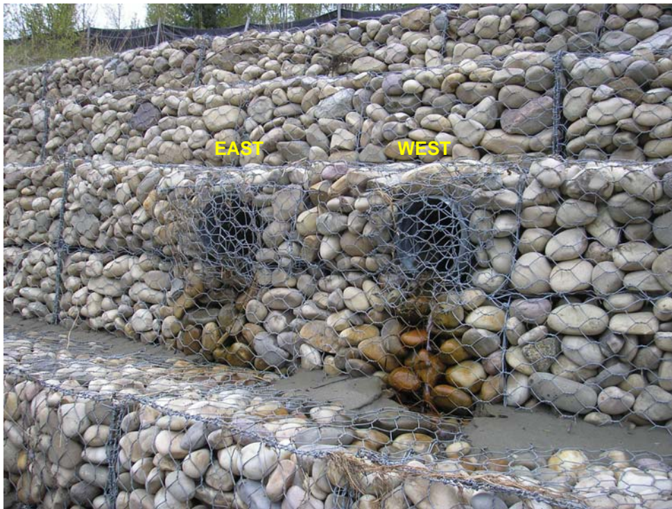
Photo 6 - Collection points east and west outlet (note that despite not currently producing water the east outlet shows signs of water stain below on the culvert).
