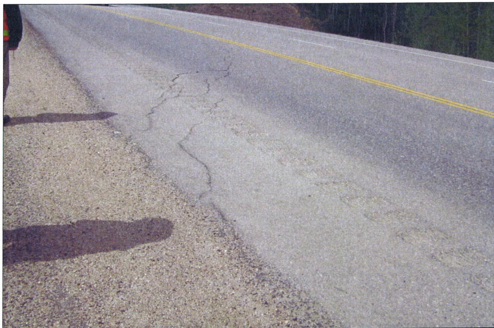
Photo 4 Pavement cracking at west flank of slide area
