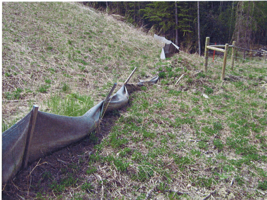
Silt fences in need of maintenance
