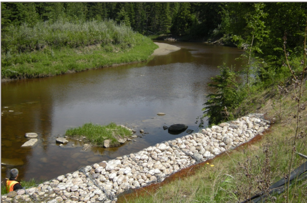
Photo 6: Gabion baskets erosion protection at Modeste Creek
