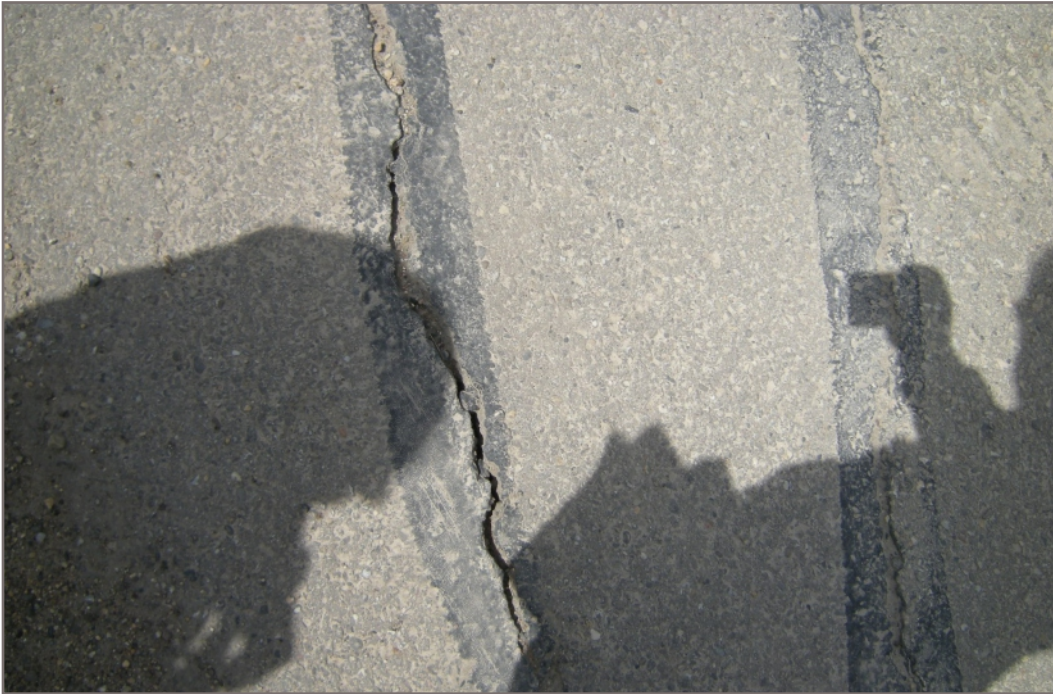
Photo 5: Pavement cracking through sealant
