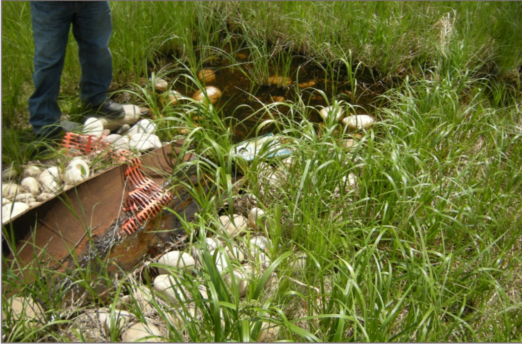
Photo 3: Inlet of culvert on east portion of slide above base of ditch
