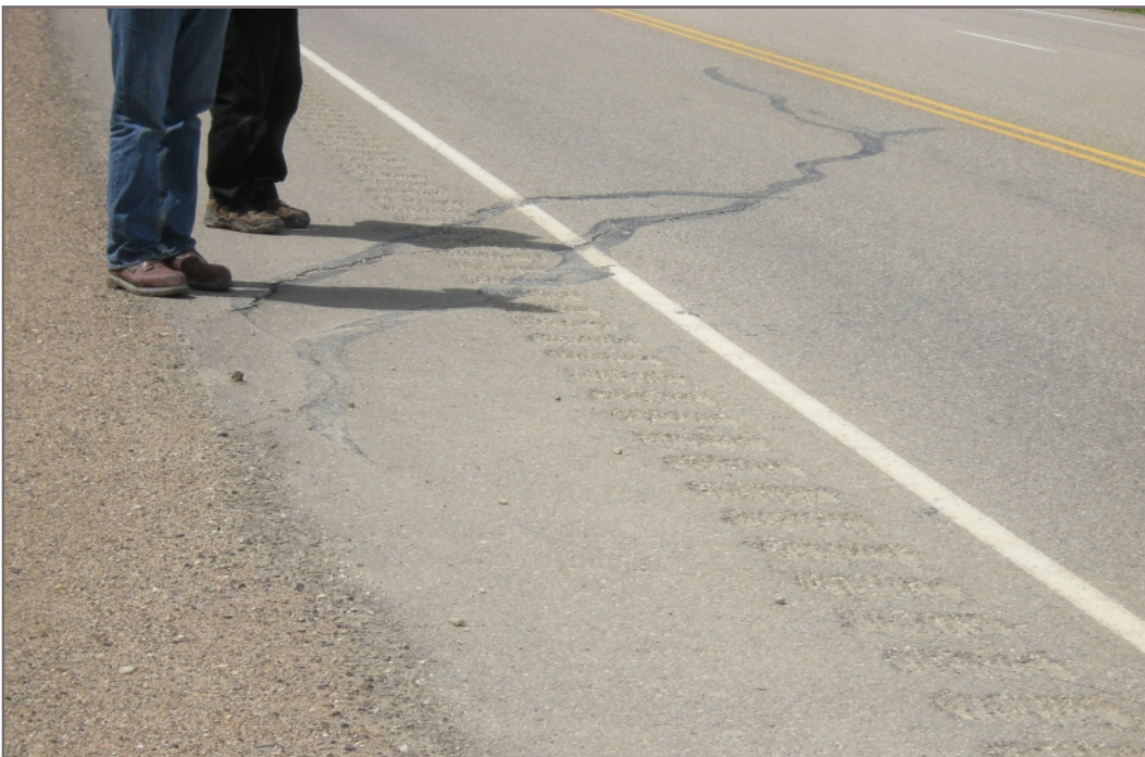
Photo 4: Pavement cracking at west flank of slide area sealed in 2010
