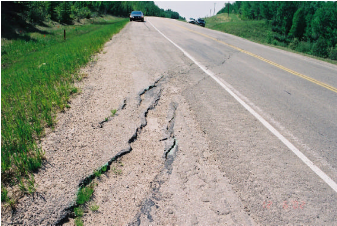
PAVEMENT DISTRESS, 20 mm DIFFERENTIAL HEIGHT (LOOKING WEST)
