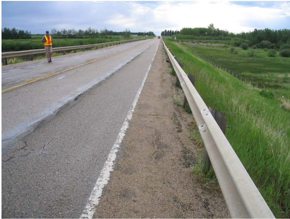
Photo 1 - Looking east at the re-aligned guard rails, June 7, 2006.
