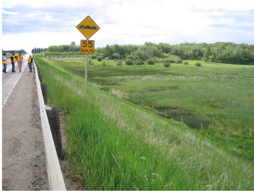
Photo 6 - Looking north at the top of north embankment slope, June 7, 2006.
