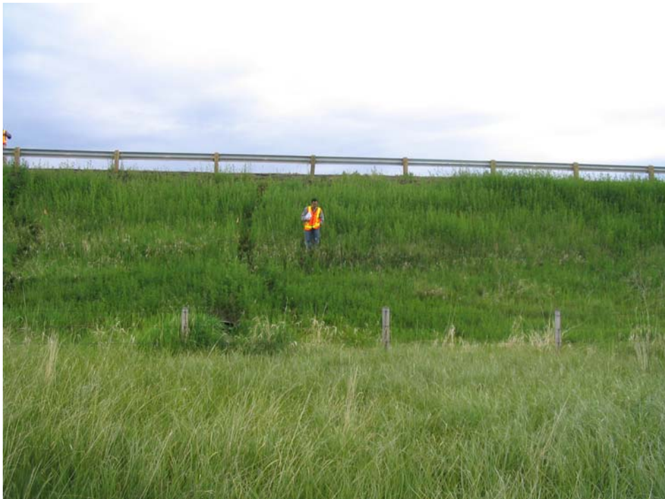
Photo 5 - Looking north at subdued shallow slump Area, June 7, 2006.
