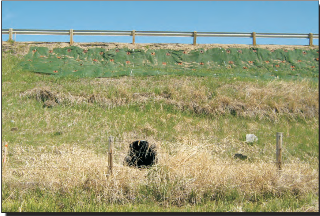
Photo 3 Profile of repaired slope
