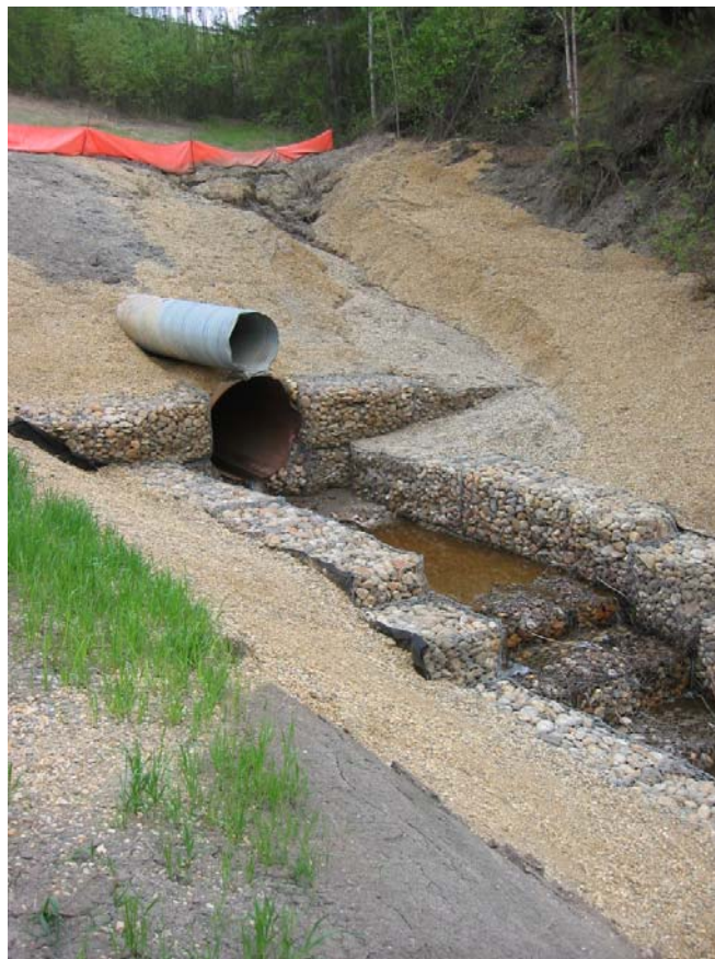
Photo 2: Whitemud River Station 42+600, repaired culvert outlet, minor erosion to be repaired, May 2003
