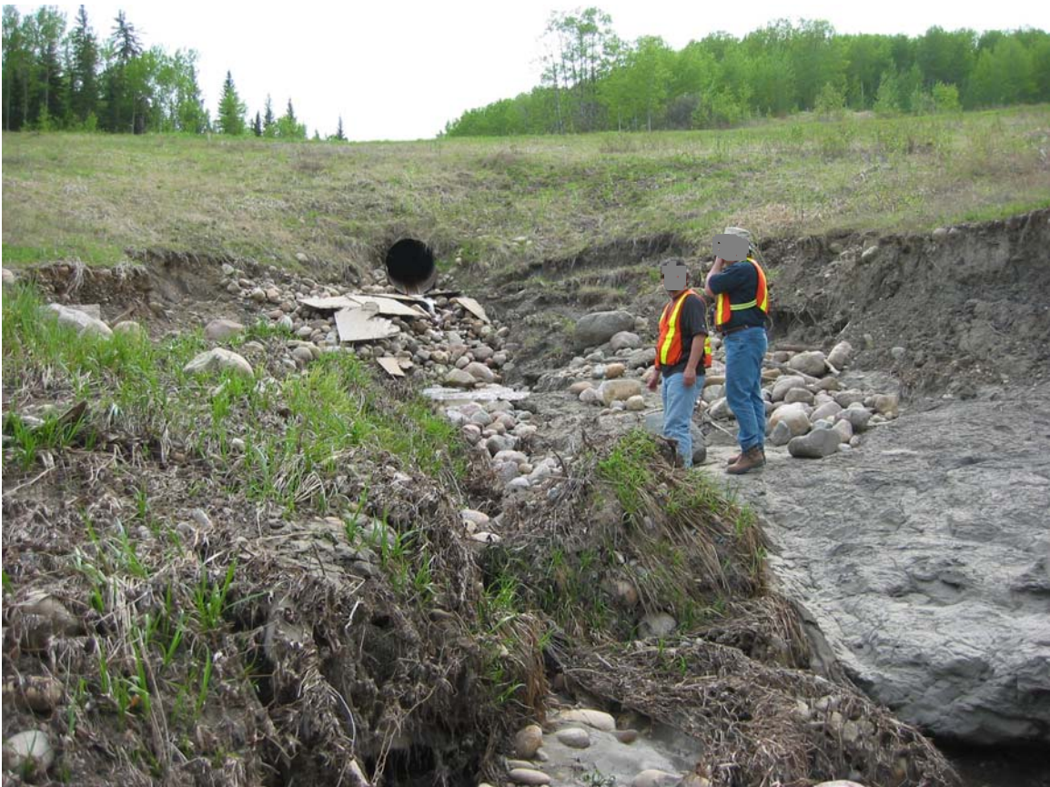
Photo 8: Whitemud River Station 44+000, erosion at culvert outlet, gabions left, shale bedrock right, May 2003
