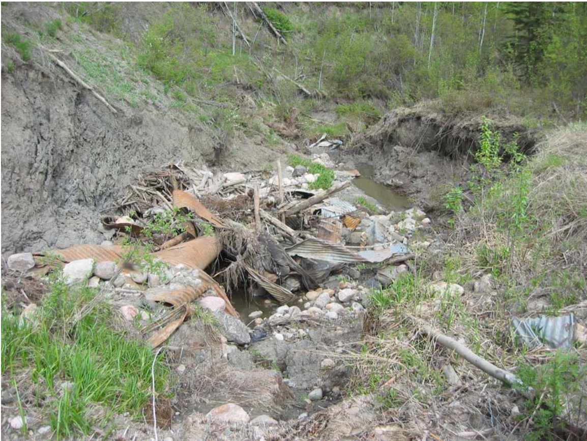
Photo 7: Whitemud River, Station 44+000, erosion downstream of culvert crossing, May 2003
