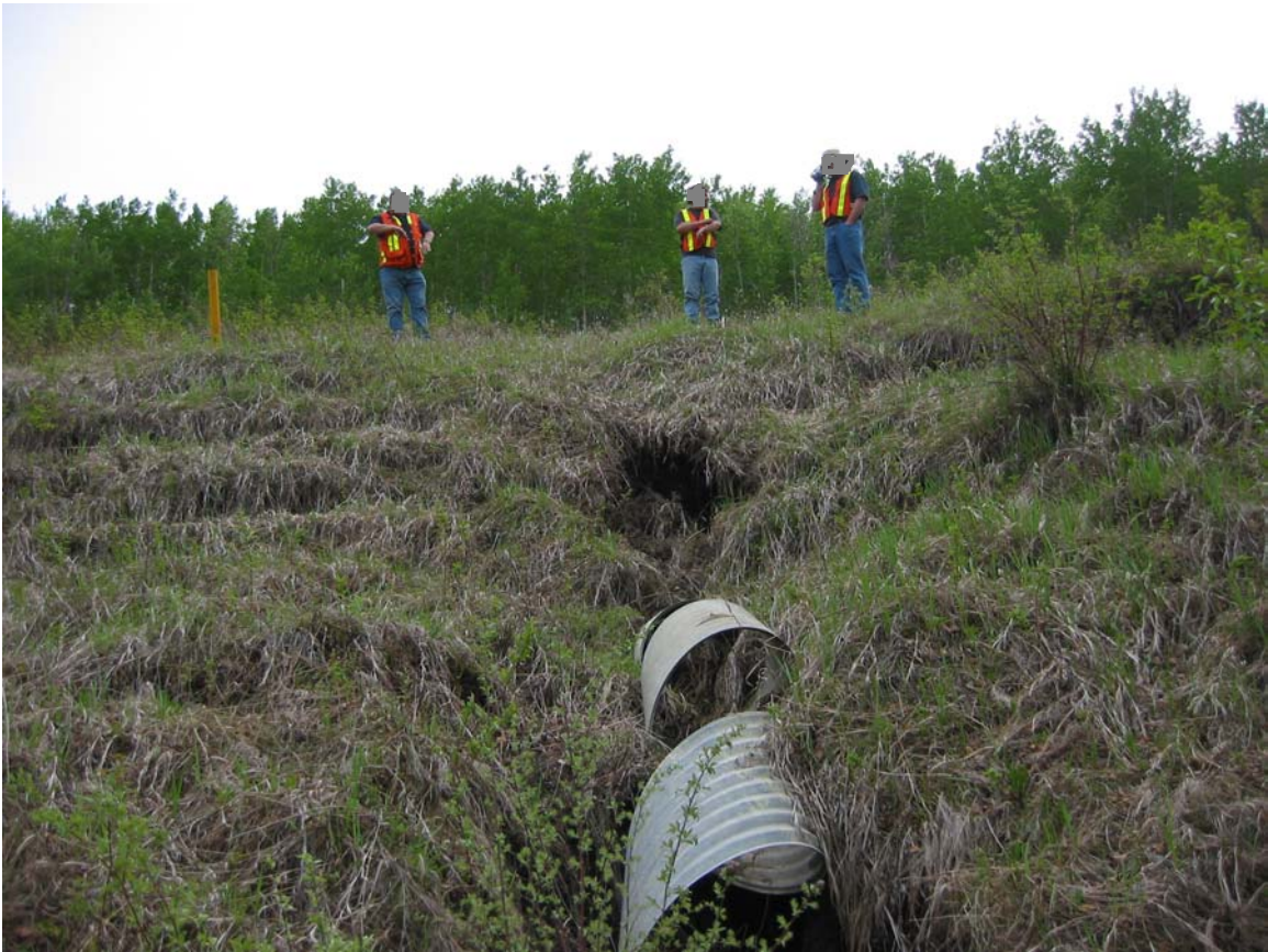
Photo 9: Whitemud River Station 45+800, slumping at culvert outlet, May 2003
