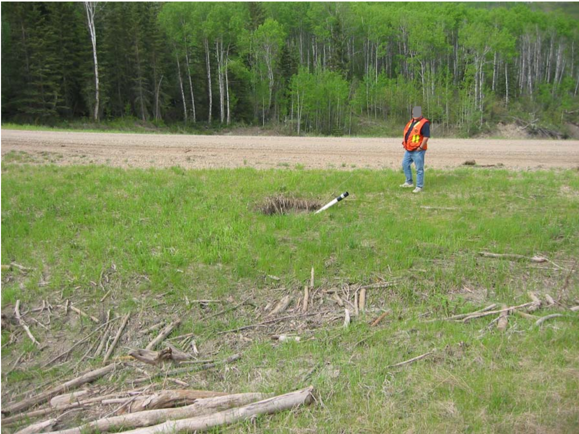
Photo 6: Whitemud River Station 44+000, sinkhole at culvert crossing, May 2003
