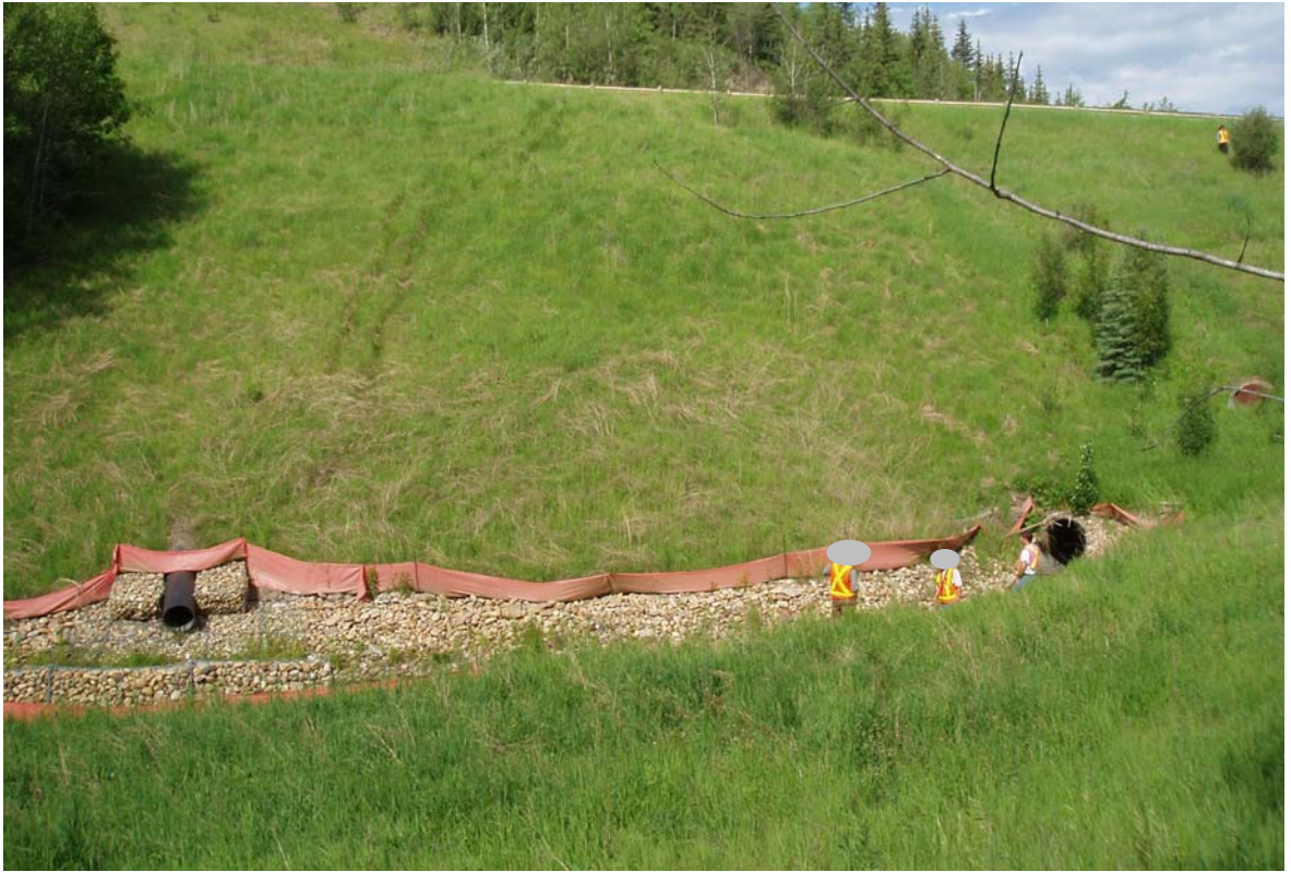
PHOTO 7: Sta. 42+600, Repaired Slope and culvert inlet
