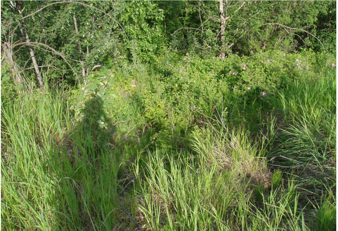
PHOTO 3: Sta. 43+200, Shallow erosion gully on the highway sideslope
