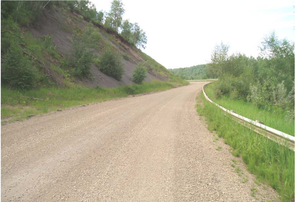
PHOTO 1: Sta. 43+200, Shale backslope looking in the SE direction
