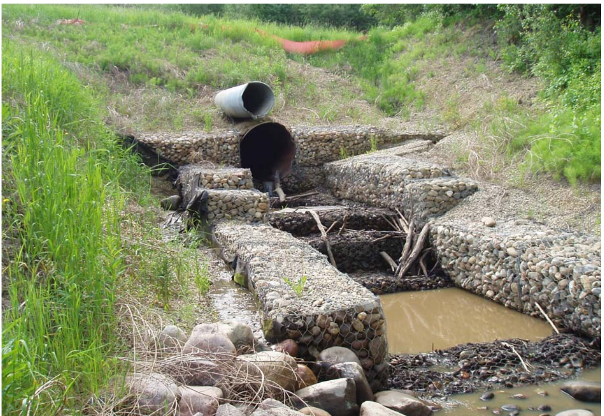
PHOTO 6: Sta. 42+600, Culvert outlet and gabion walls
