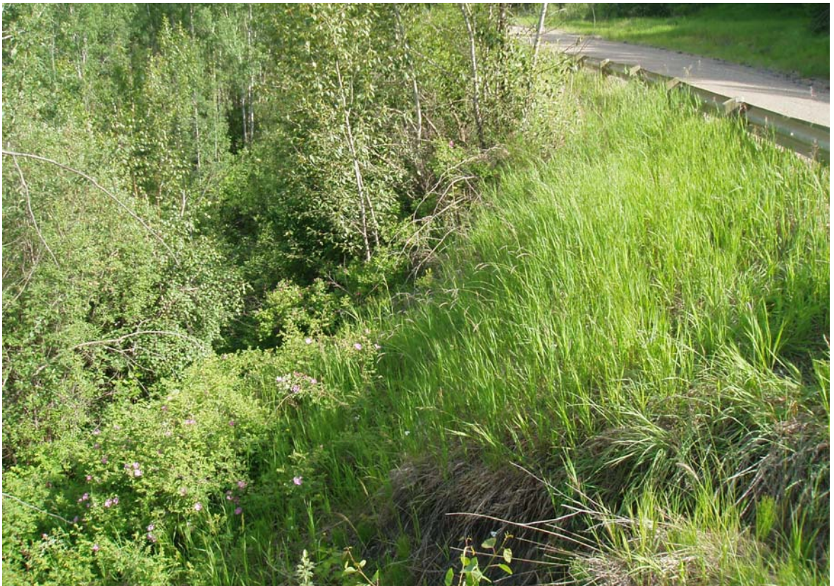
PHOTO 4: Sta. 43+200, Highway sideslope
