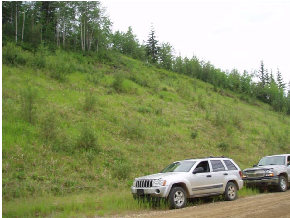
Photo 3 – Shallow slides in cut slope in the west side of highway at Station 42+600, June 16, 2006.
