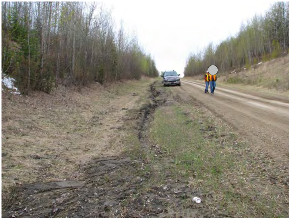
Photo 4 - Ditch erosion, looking south.
