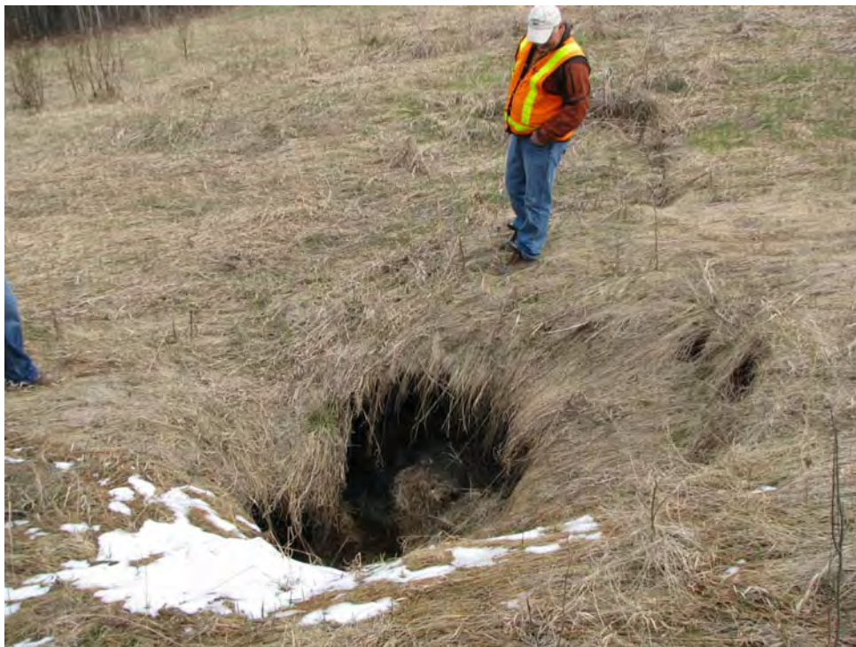
Photo 2 - Sinkhole on the west slope, near the culvert alignment.
