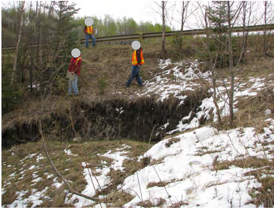
Photo 3 - New slump on the west sideslope, looking east.
