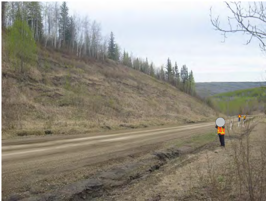
Photo 5 - View of shallow backslope failures at the south end of the site, looking northwest.
