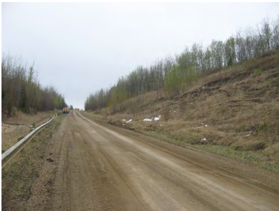
Photo 6 - Backslope failures on the west side of the highway, looking southwest.
